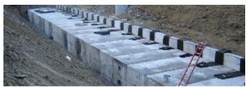
Confined space entry and inspection of BMP system -City Public Works staff performed entry and inspection with guidance/feedback from OHM Advisors staff. This includes sediment measurement in "solid" chambers, sediment measurement in the "infiltration" portion, and measurement of sediment migration across the "infiltration" portion of both systems.
