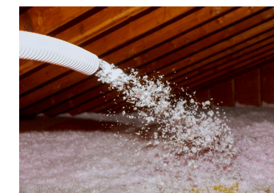
Insulation added to attic space
