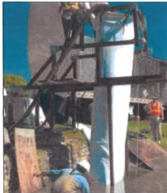
Subaqueous installation of CIPP into storm drain
