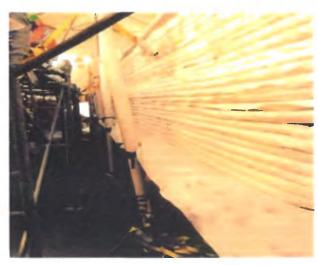
rehabilitation of sanitary sewers using the Cured-In Place pipe lining method. Work under this contract included 4,350 LF of 48" sanitary sewer located along Haggerty Road and Joy Road pavement. The 4,350 LF project included bypass, pipe cleaning and CCTV in addition to the over the hole CIPP liner installations.
