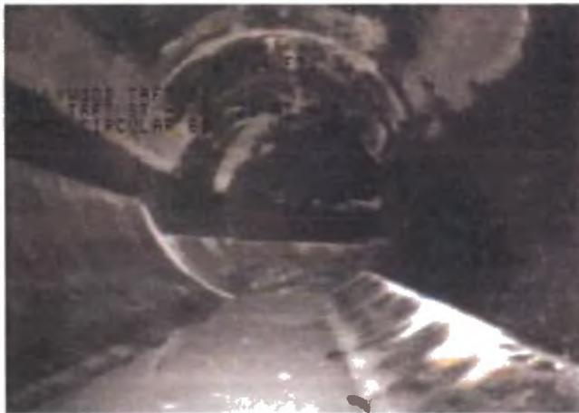
Lanzo Trenchless Technologies was the prime contractor for this project and self-performed most of the work associated. The project included obtaining permits associated with the project, traffic control and cleaning and CCTV investigation of the sewers, Cured-In-Place Pipe rehabilitation, point repairs, grouting & other incidental work. After review of the videos, Lanzo designed the liner tubes per ASTM specifications
