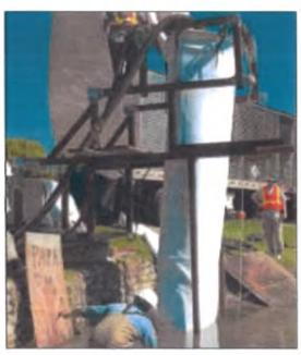
Subaqueous installation of CIPP into storm drain
