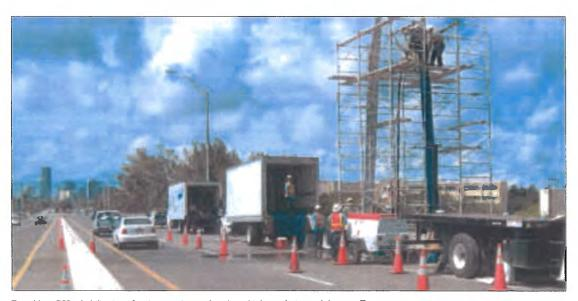
Trenchless CIPP rehabilitation of a pipe running under a busy highway during rush hour traffic
