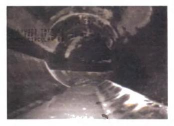
Lanzo Trenchless Technologies was the prime contractor for this project and self-performed most of the work associated. The project included obtaining permits associated with the project, traffic control and cleaning and CCTV investigation of the sewers, Cured-In-Place Pipe rehabilitation, point repairs, grouting & other incidental work. After review of the videos, Lanzo designed the liner tubes per ASTM specifications
