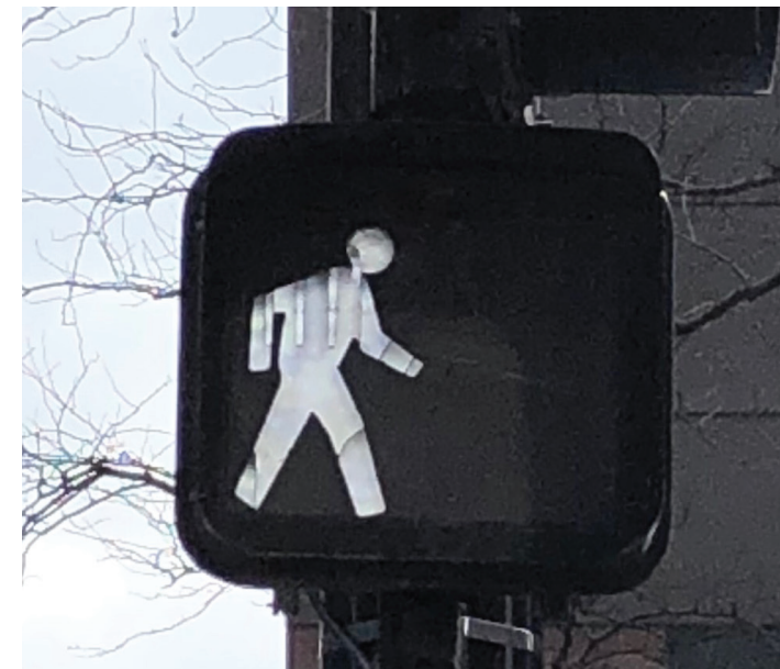
Pedestrian Signal Head in Chicago, IL
