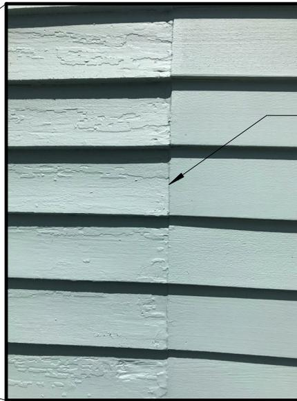
Seam in siding on South Elevation showing location of infilled porch.
