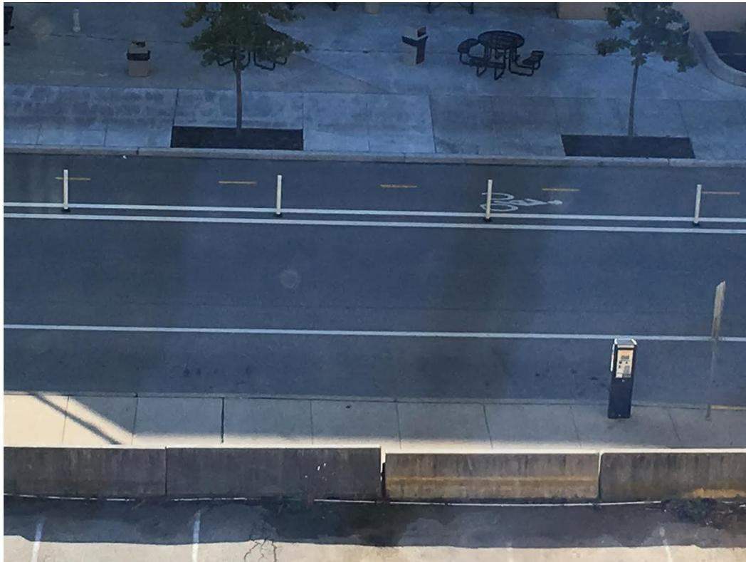
I didn't take exhaustive notes or measurements, but notice that the buffer is relatively narrow - possibly 1' - but the vertical pylons add significant protection nonetheless (FWIW: this street appears to have 1 curbside parking lane, 1 vehicle lane, and the 2-way protected bike lane).
