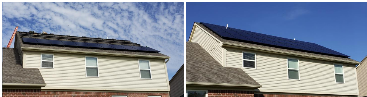
Solar panel installation on shingle roof
