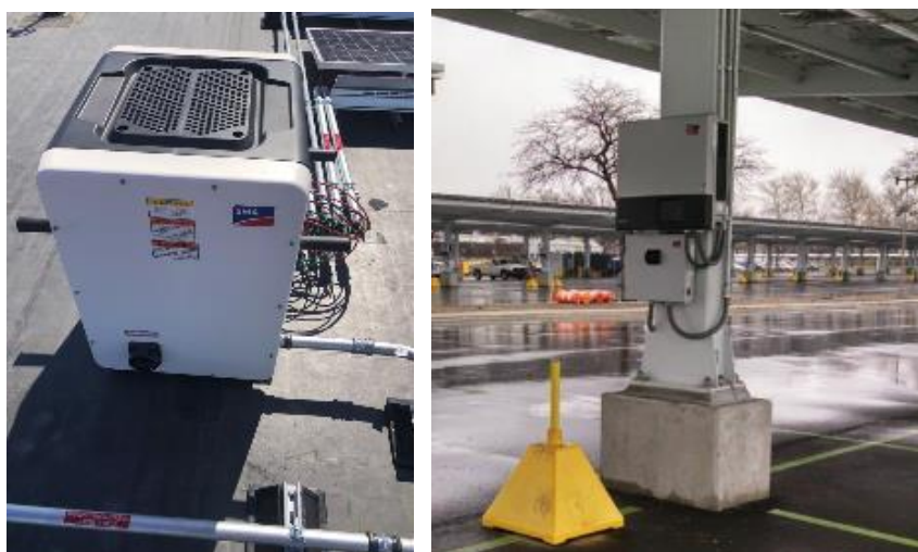
Examples of inverter on roof and mounted on column
