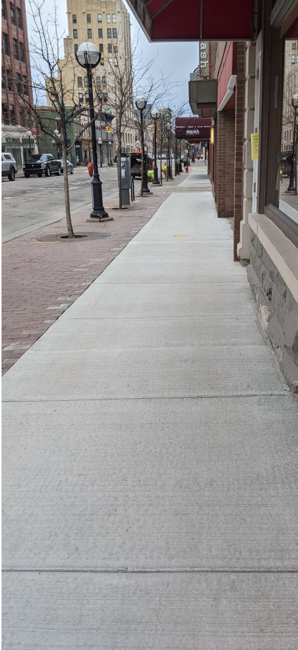
Sidewalk and Paver Repair
