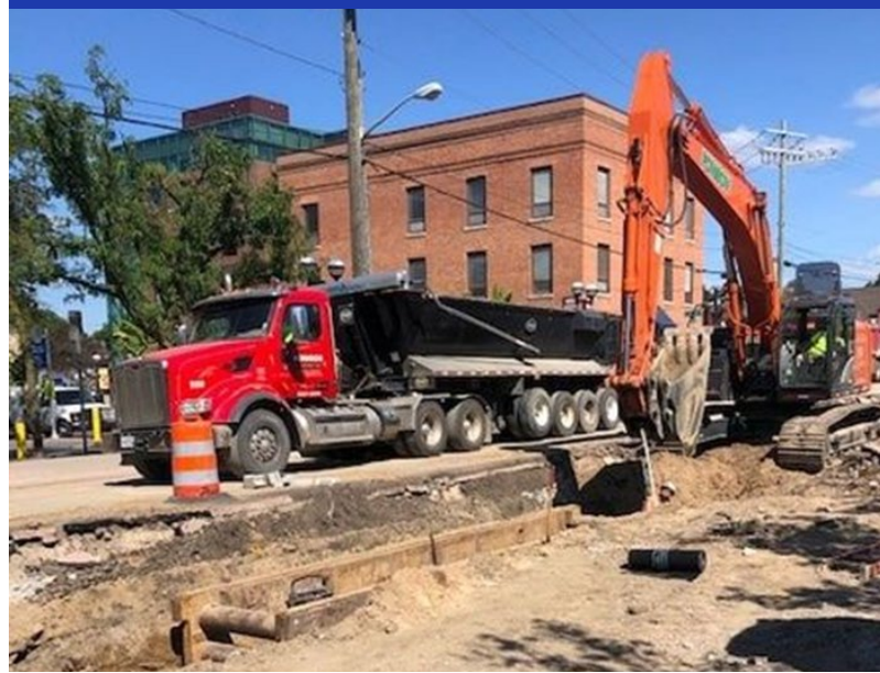
Miller/Catherine AAHC Utility Work (2022)
