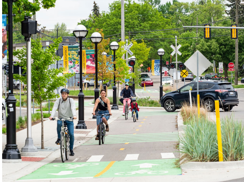
First Street Reconstruction (2021)
