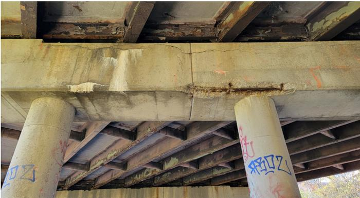
The project special provision for Structural Steel Galvanizing indicates the existing beams are to be removed, salvaged, cleaned, repaired, and sent to a facility for placement of galvanized coatings to match the proposed new beams.
