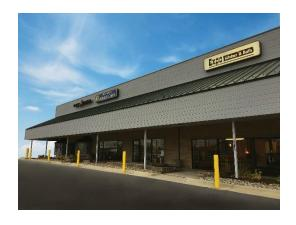
Westgate Shopping Center is home to one of the oldest outdoor malls in Ann Arbor. This project consisted of the structural and aesthetic renovation of the 1400 lineal feet of canopy for Westgate including new siding, sheathing, canopy lights, and new columns. Safety was a primary concern as businesses remained open, we worked closely with the owner and tenants to advise a plan that entailed the utmost safety measures for employees and customers.
