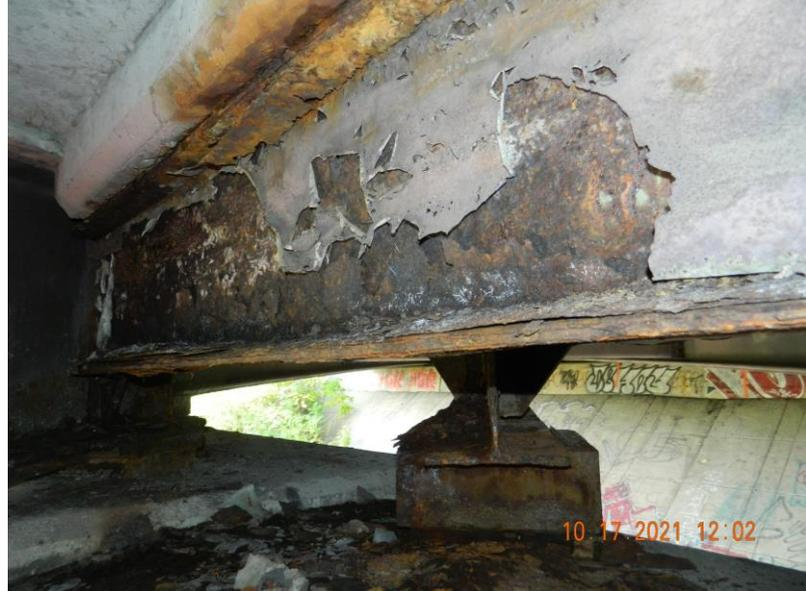
Photo 4: Typical Beam End with Paint System Failure and Section Loss
