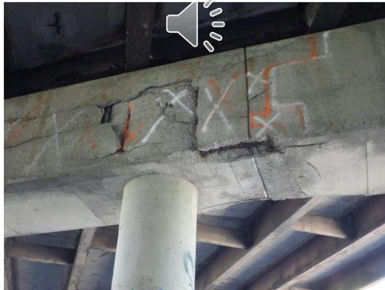
Photo 3: Spalled Pier Cap with Exposed Rebar
