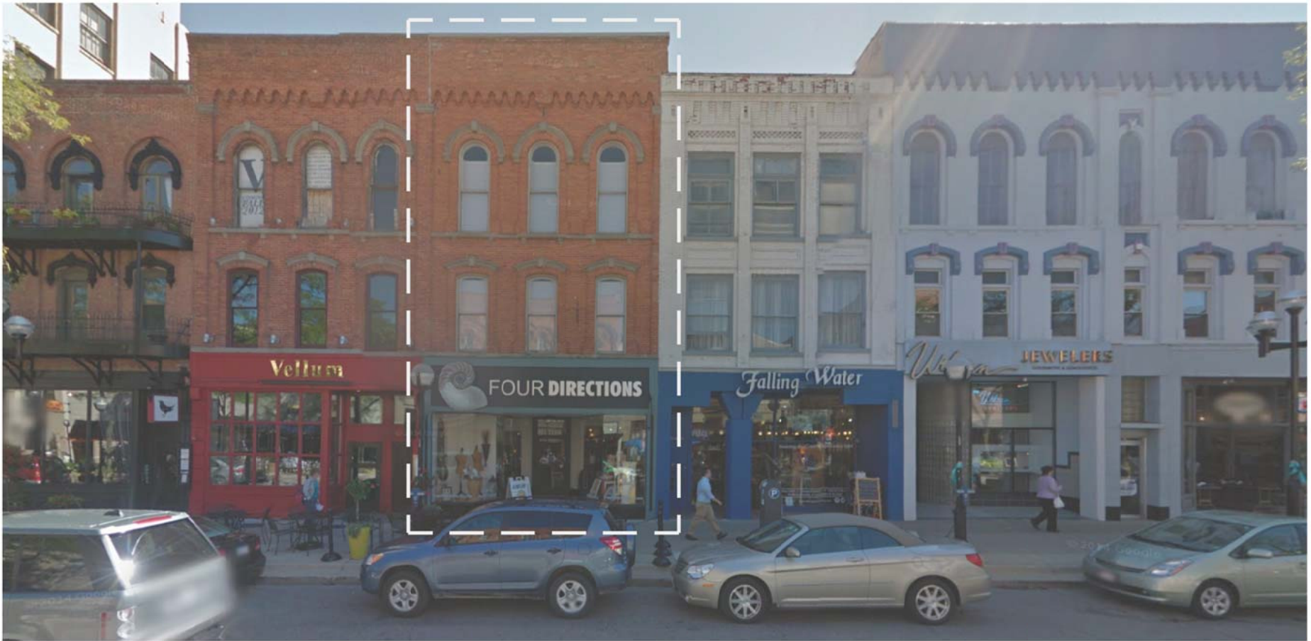
EXISTING CONDITIONS, VIEW FROM WEST (MAIN STREET)
