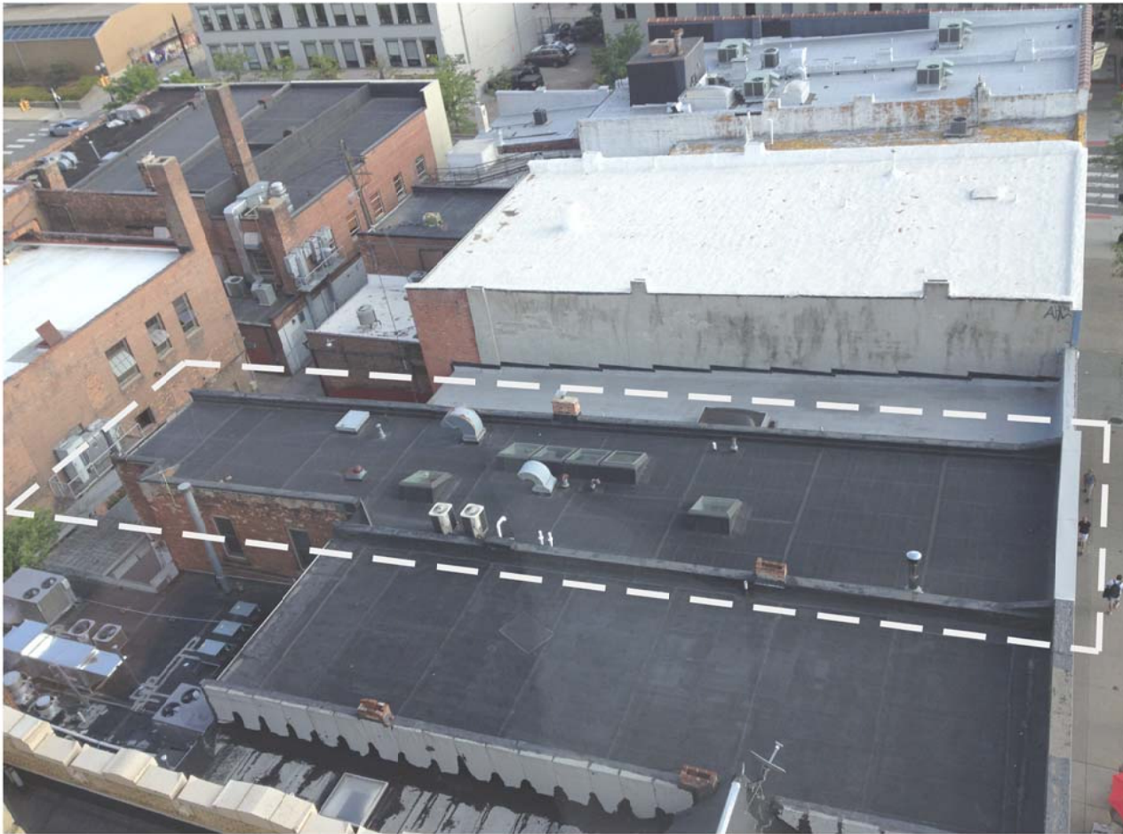
EXISTING CONDITIONS, VIEW FROM NORTH (ROOF)
