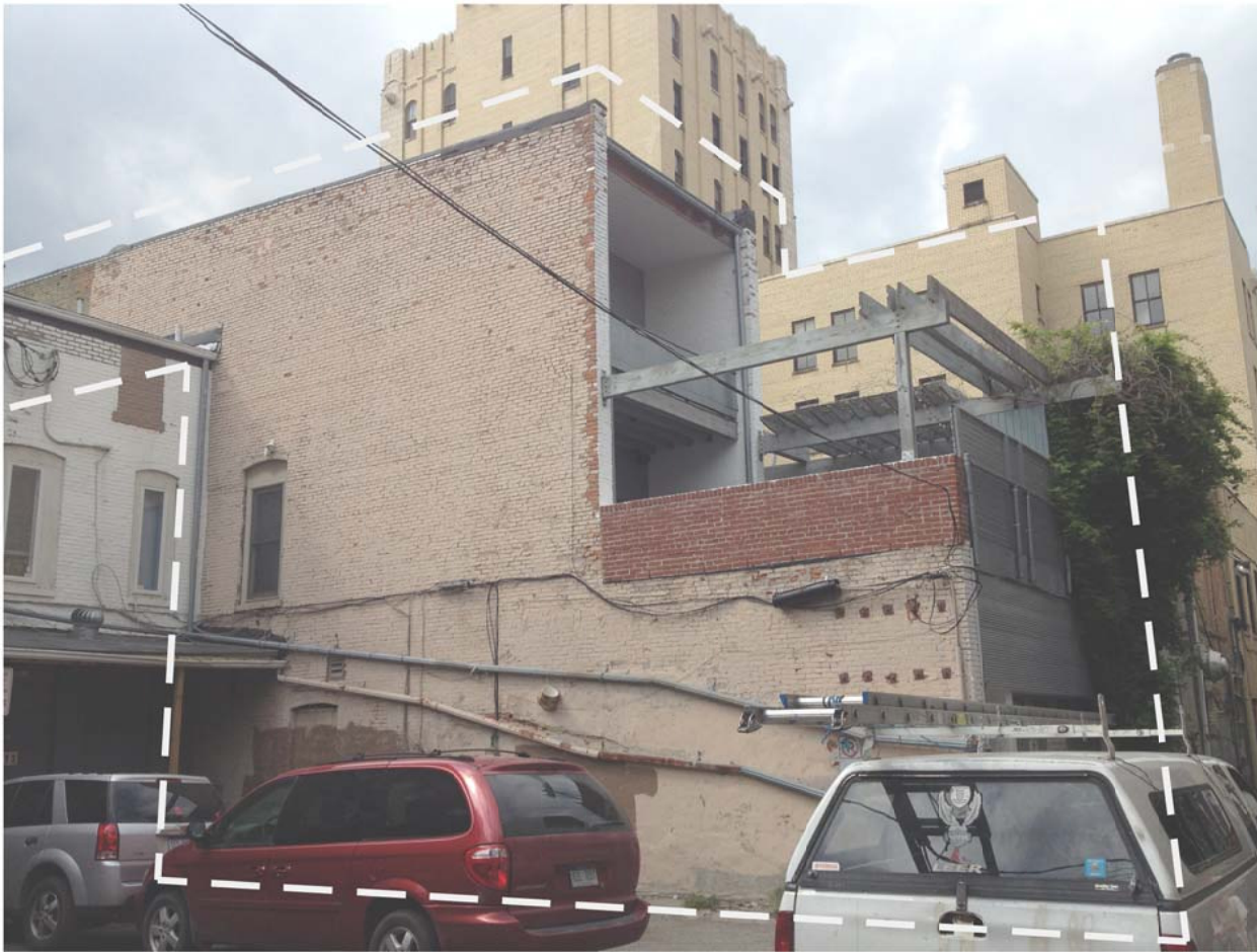
EXISTING CONDITIONS, VIEW FROM SOUTHEAST (ALLEY)
