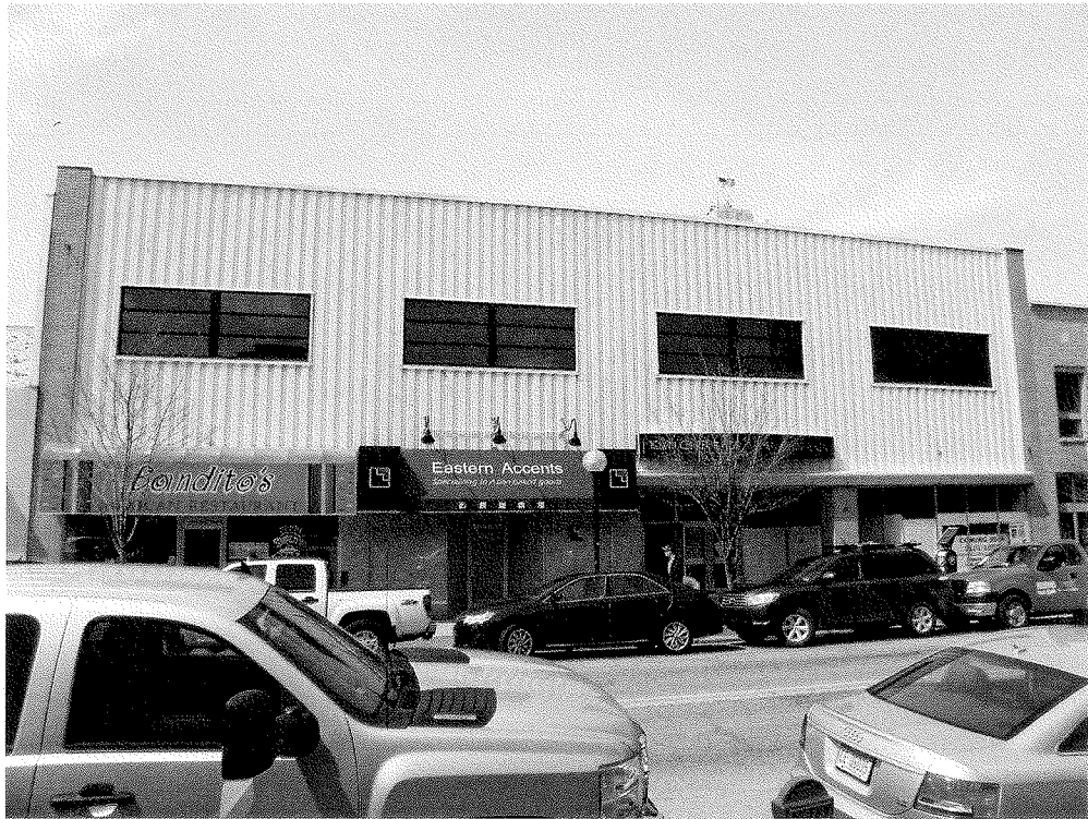
Existing Eastern Facade 210-216 S 4th Ave.
