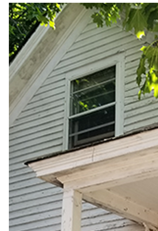
Existing window - DH-C
