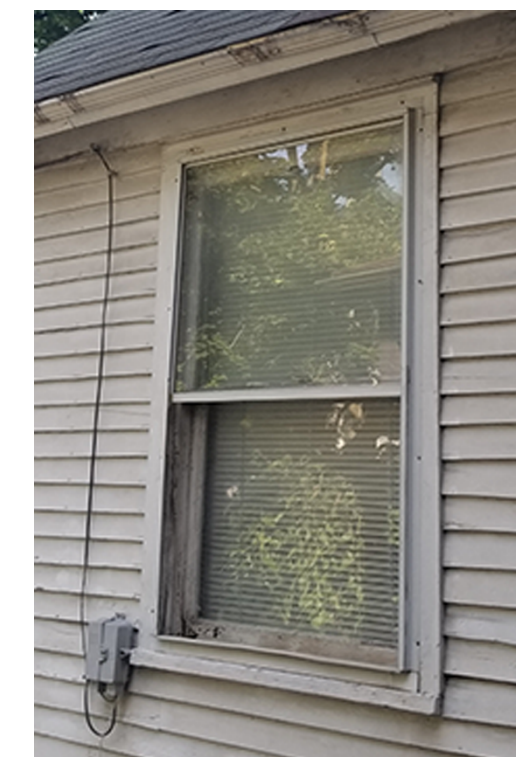
Existing window - DH-A
