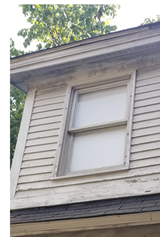
Existing window - DH-B
