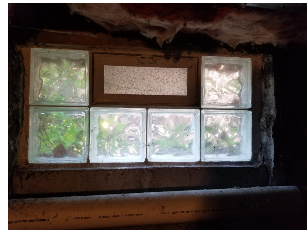
Existing window - GB-A
