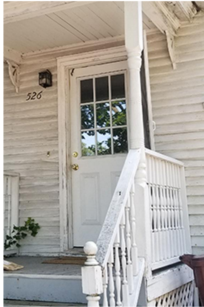
Existing front door
