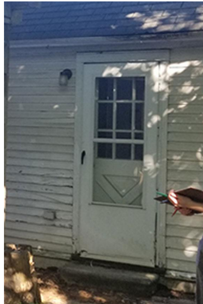
Existing back door - TO BE REMOVED AND INFILLED
