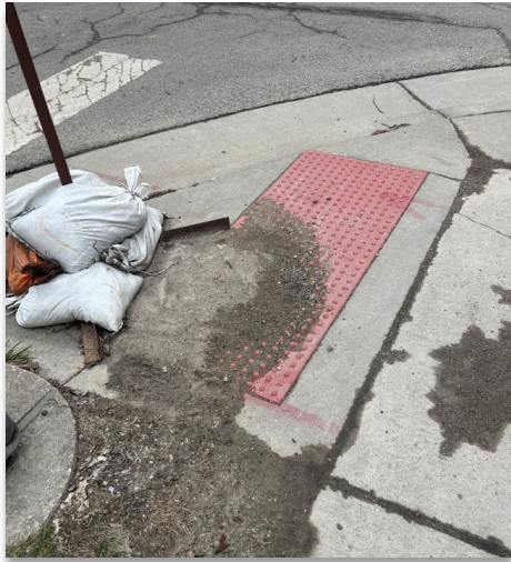
Figure 18 - ADA Compliance Issues at Intersection Corners
