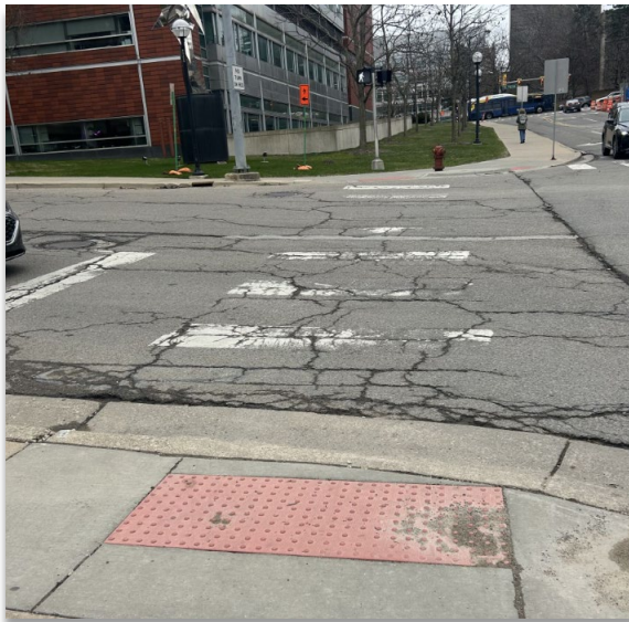
Glen Ave and Ann St East Leg Stop Bar and Crosswalk
