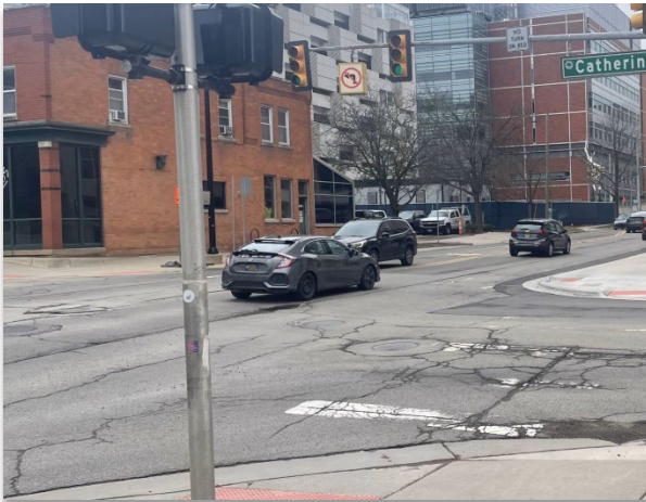
Southbound Approach at Glen Avenue and Catherine Street
