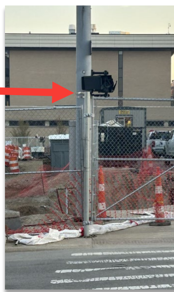
Broken Pedestrian Signal Head, Northwest Corner
