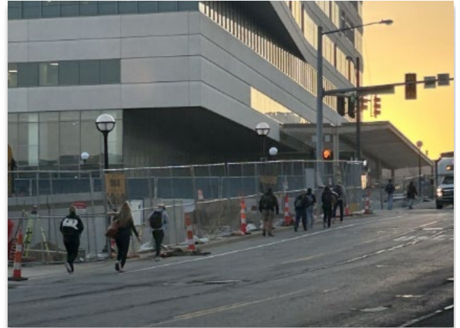
Pedestrians Walking in the Road Along the Closed Sidewalk on Ann Street
