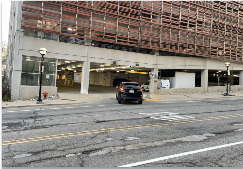
Figure 23 - Improper Left Turn into Ann Street Parking Garage
