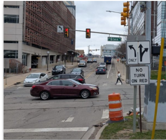
Eastbound Approach at Glen Avenue and Ann Street
