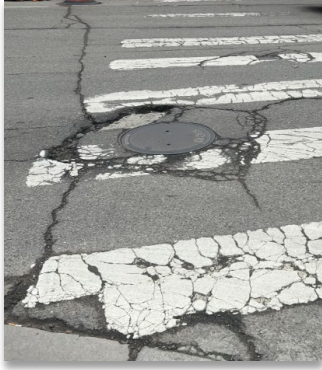
Cracked Pavement Throughout the Study Area
