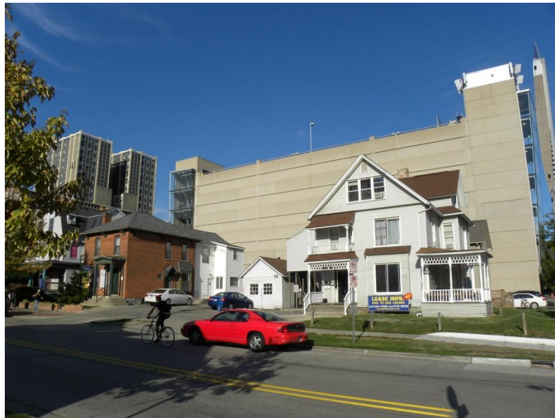
Western face of Forest St. Parking Structure
