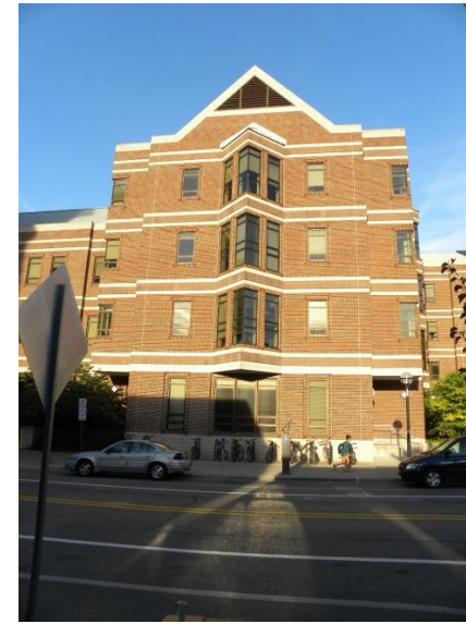
Adjacent U of M building on E. University
