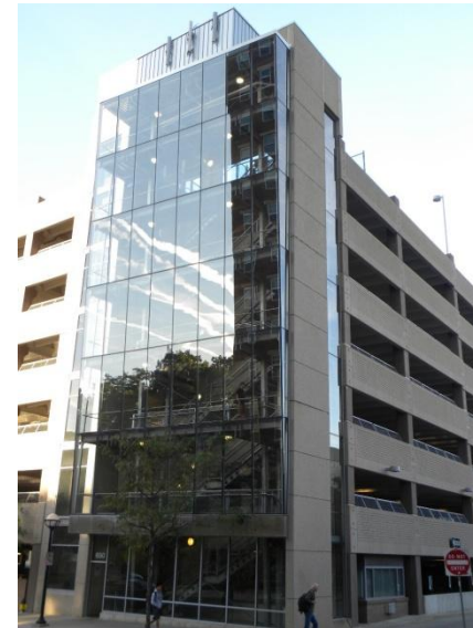
Stair tower at the Forest St. Parking Structure
