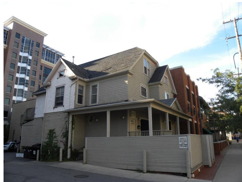
Existing residential structure to be demolished
