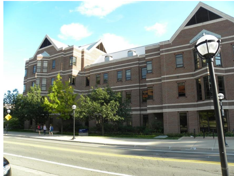
Adjacent U of M building on S. University
