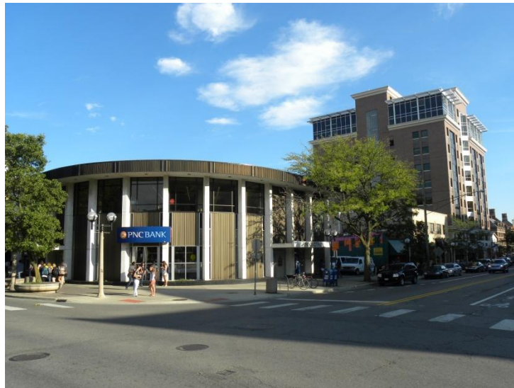
PNC Bank on the SE corner of S. and E. University Streets with Zaragon Place in the background.
