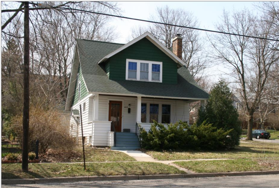
617 W Madison Street (2008 Survey Photos)
