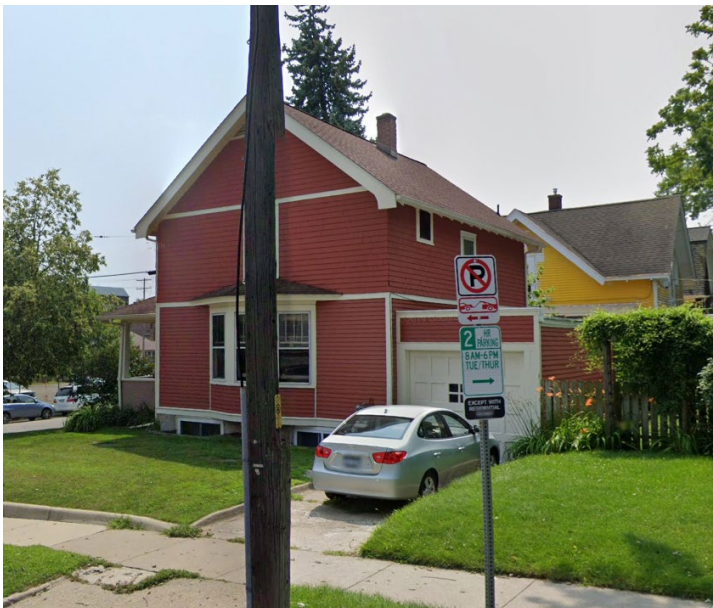
Chimney (courtesy Google Street View 2019)
