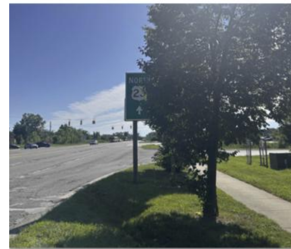
Vegetation Obstructing Signage
