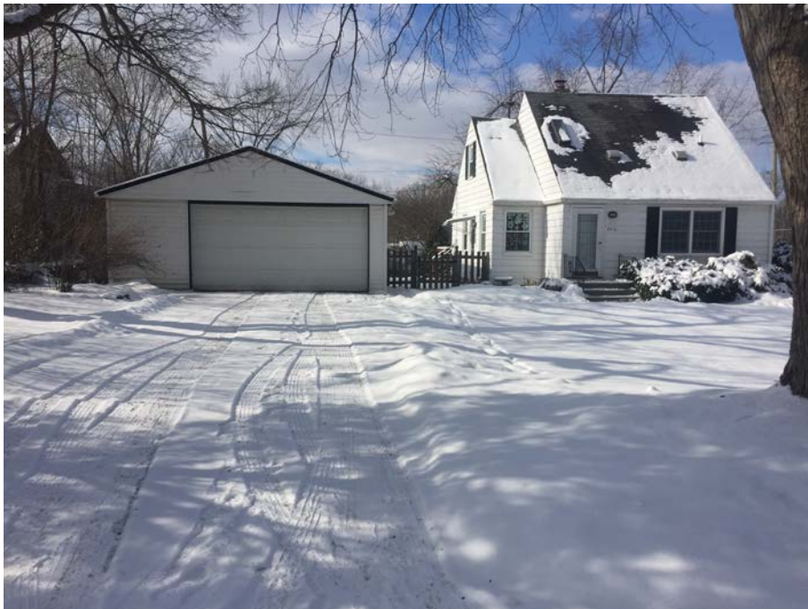
Front view of McDaniel House from Elmwood curb. Only adjoining neighbor is to the left of garage. NOTE: New porch will occupy about the same space as current concrete stoop and giant shrubs
