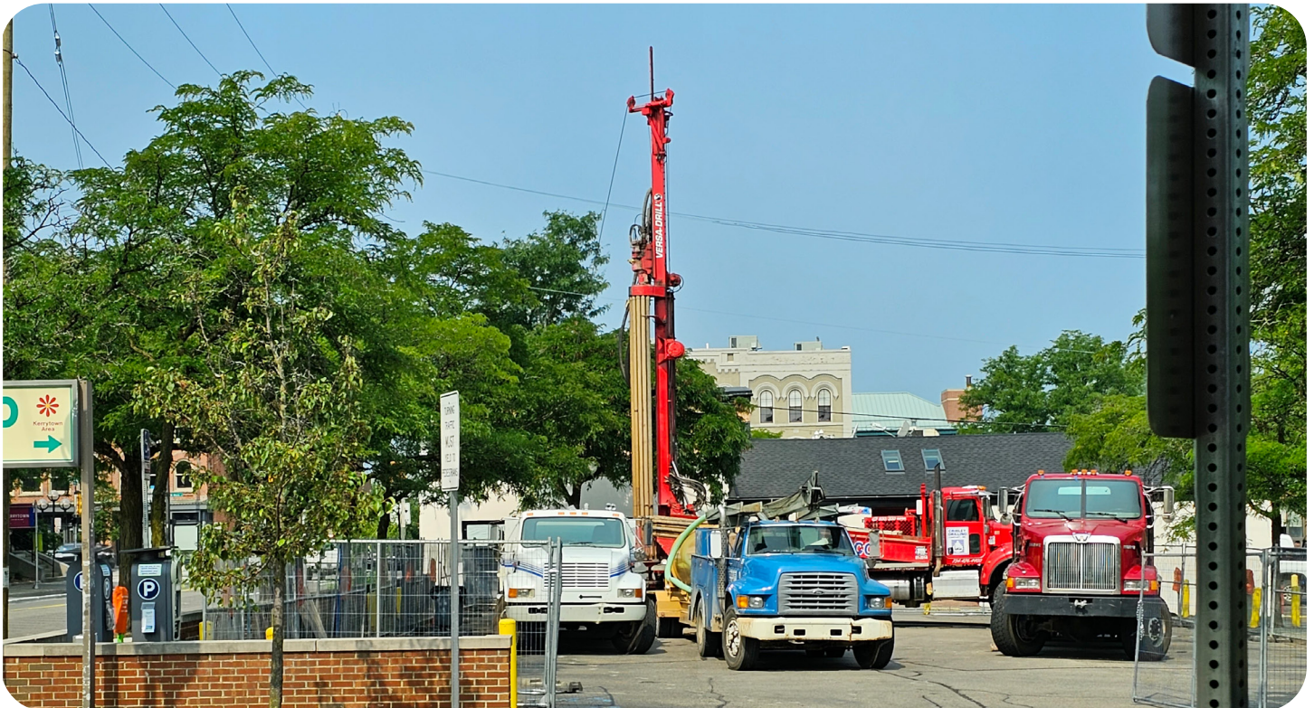
Drilling for the installation of geothermal at 121 Catherine Street, July 2023.
