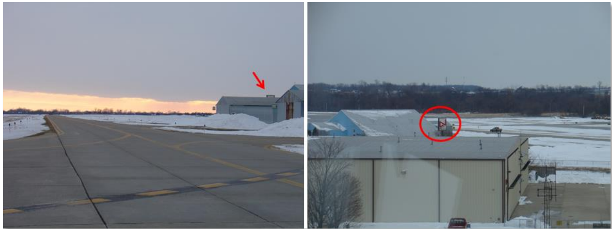
Figure 2. (L) A view from the runway looking at the obstructed control tower, (R) A view from the control tower looking at the obstructed runway.
