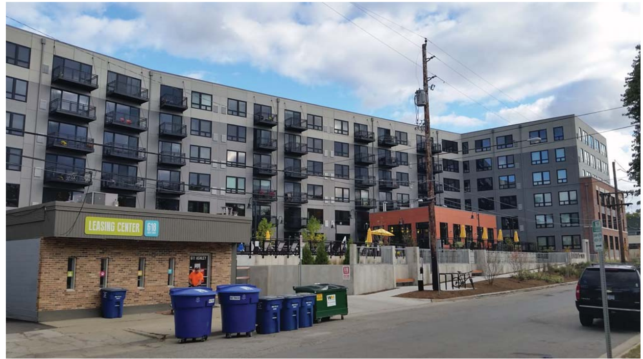
West side of 618 South Main Street Loft Apartment building between Mosley and Madison
