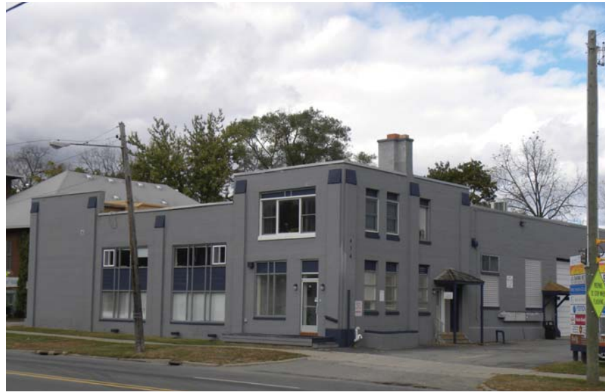
Older Building adapted for new use as offices
