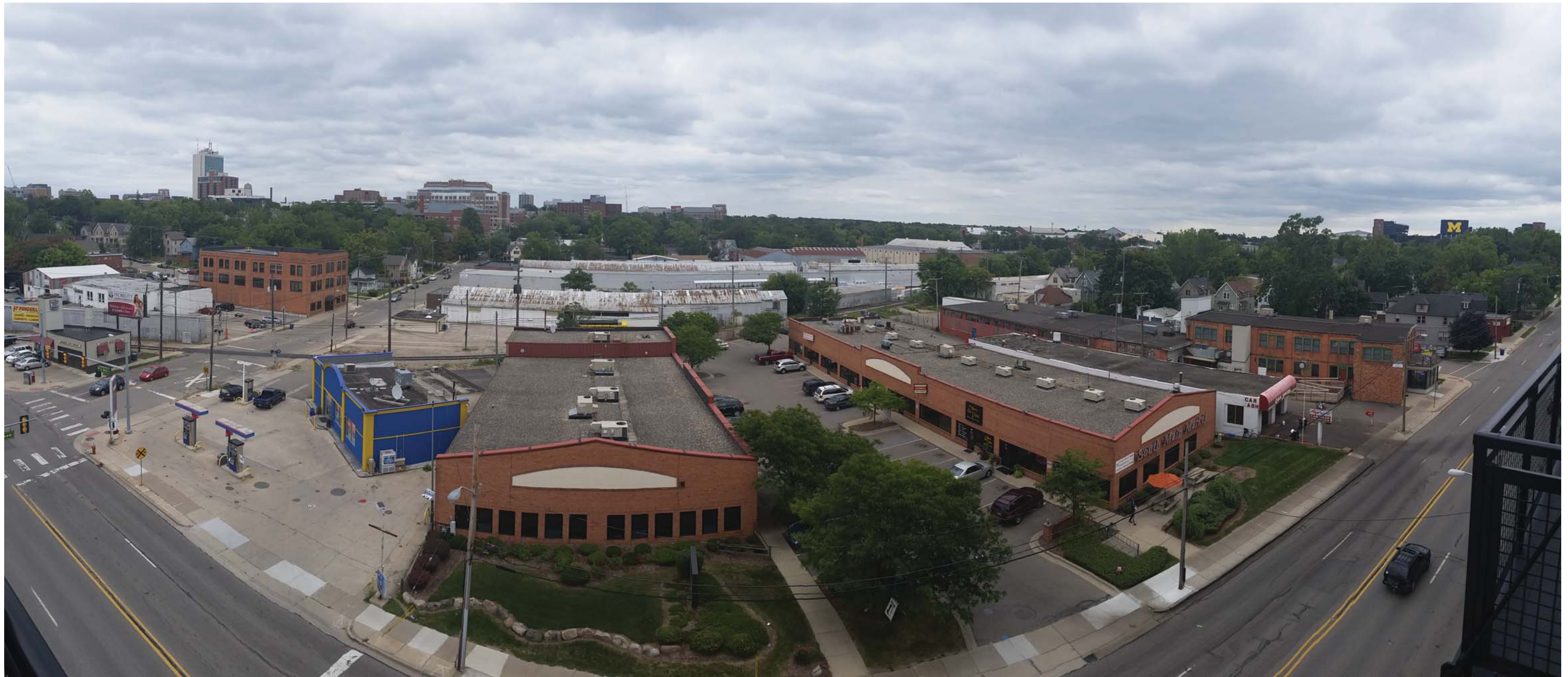
Elevated view of site looking east
