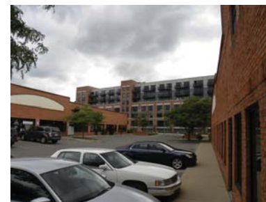
North end of site looking due west
