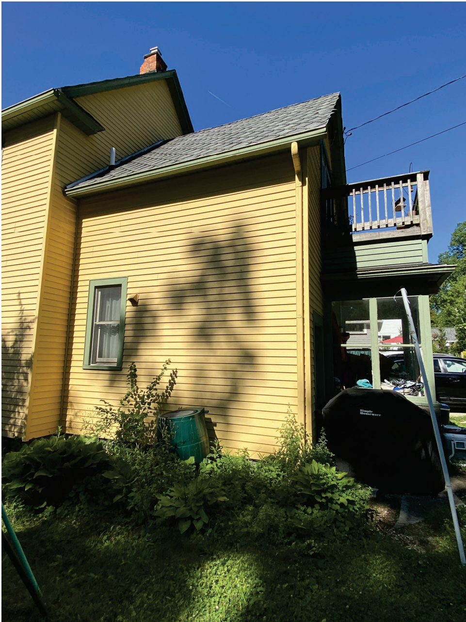
Northeast Corner of House
