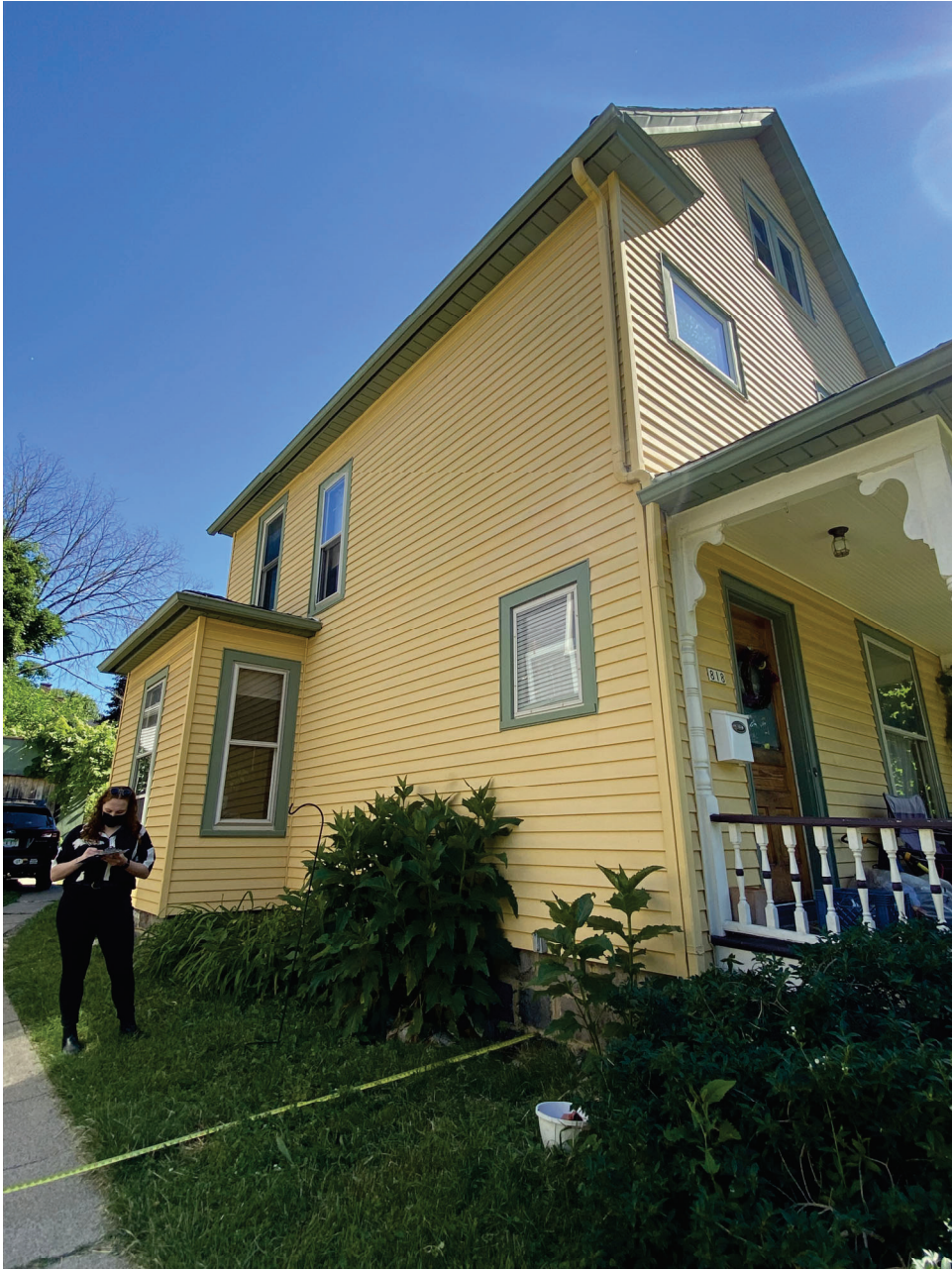
Southwest Corner of House
