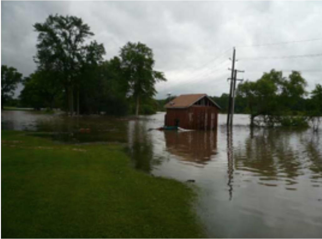
C. Pump house for Huron Hills Golf Course next to South Pond. Water in this picture is 6-7 feet above normal height of South Pond. The water had receded a fair amount before I ventured out to take this picture. (Storm of ~June 6, 2010)
