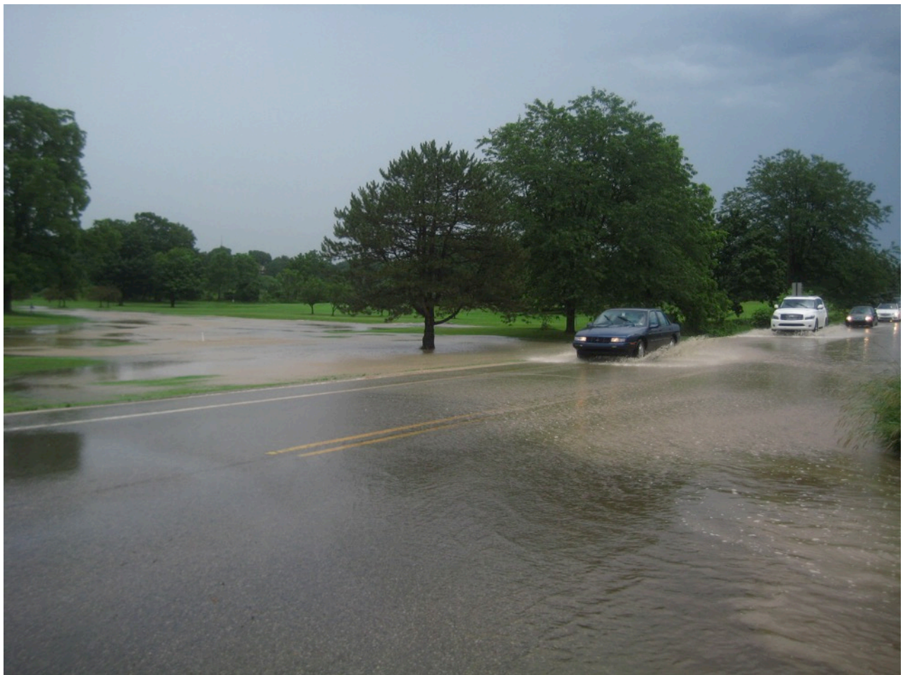
A. E Huron River Dr. just east of Elmwood looking across towards Huron Hills Golf course. The 26 inch culvert under E Huron River Drive has flooded. (Picture taken after the rainstorm had passed, ~June 28, 2013)
