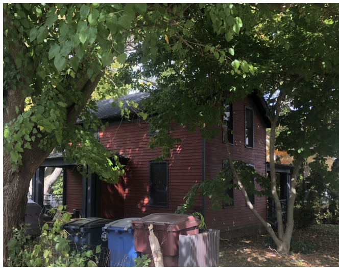
EXISTING CONDITION - PHOTO VIEW OF KITCHEN SIDE DOOR FROM SIDEWALK
