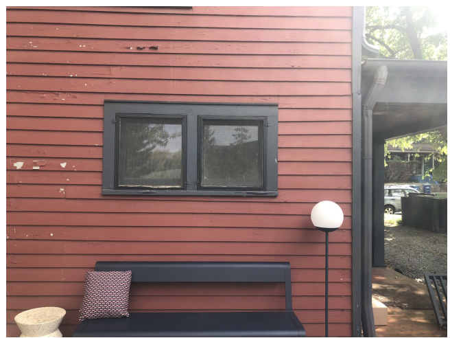
EXISTING CONDITION - PHOTO VIEW OF PROPOSED WINDOWS TO BE REMOVED
