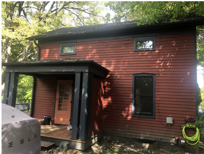
EXISTING CONDITION - PHOTO VIEW OF KITCHEN SIDE DOOR FROM DRIVEWAY
