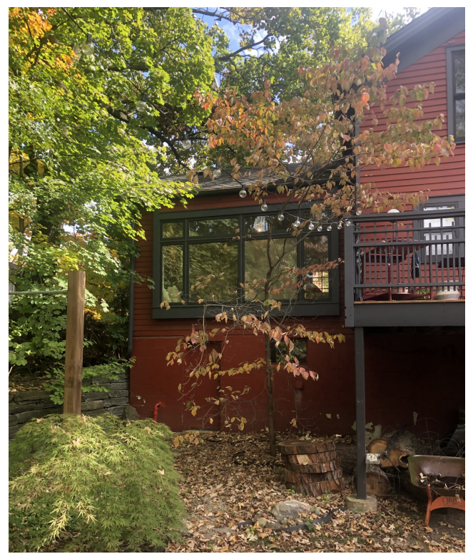
EXISTING CONDITION - PHOTO VIEW OF PROPOSED REAR ADDITION AREA
