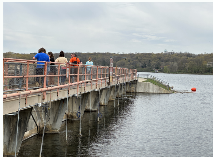
Infrastructure along the Huron River raw water source
