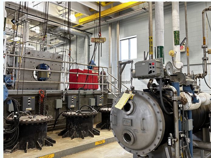
Interior of the ozone building at the water treatment plant
