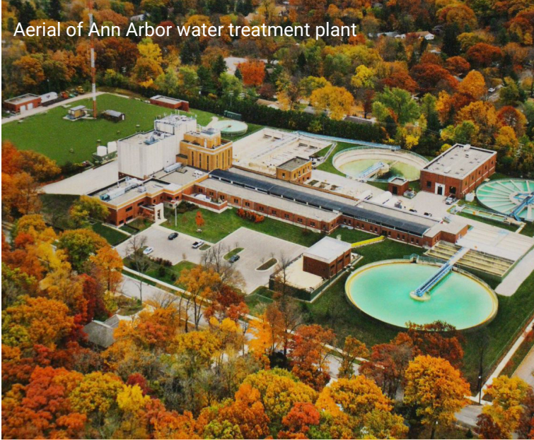
Ann Arbor water treatment plant
