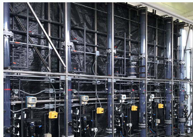
Pilot testing with filter columns to assess PFAS removal
