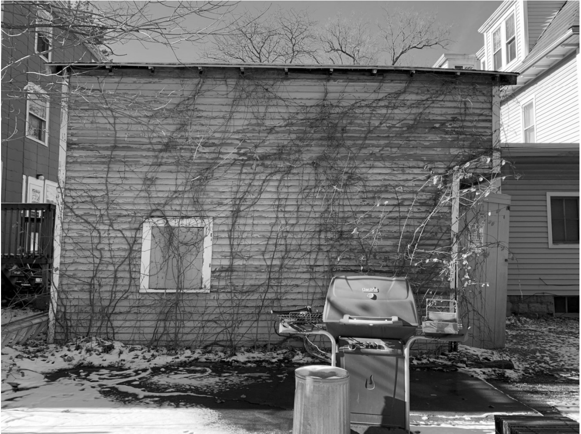
PHOTO #3 – EAST ELEVATION
