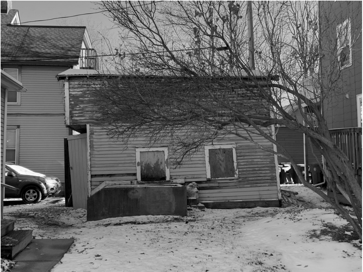
PHOTO #2 – WEST ELEVATION
