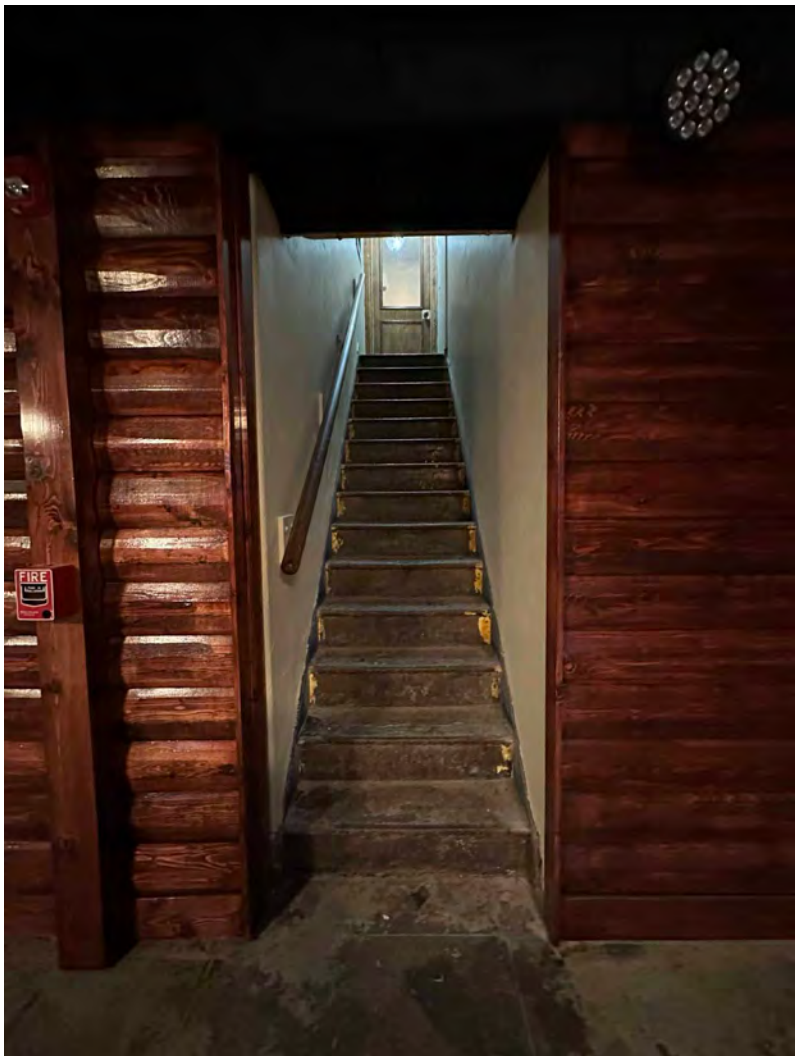
3 VIEW 3 A5.1 View up existing stairs from basement
