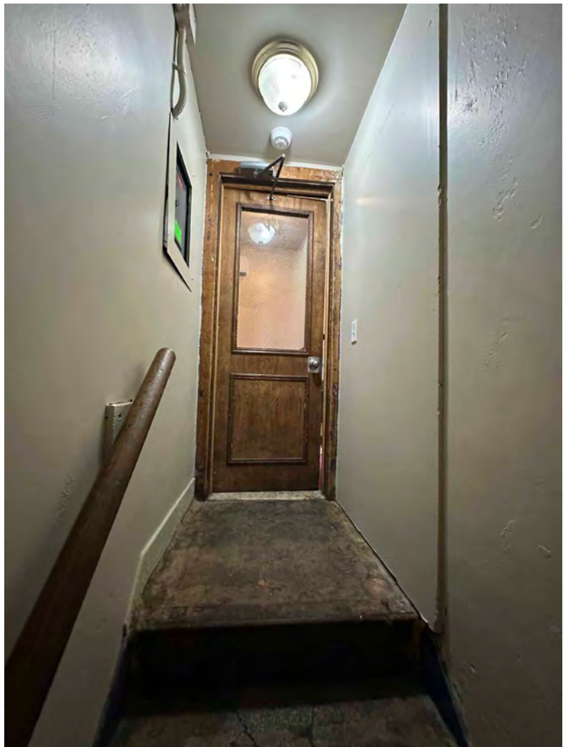
2 VIEW 2 A5.1 View of existing stairs towards stairwell door
