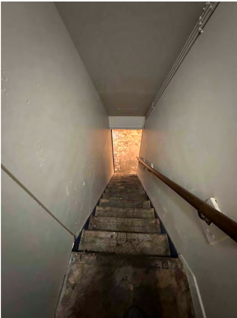
1 VIEW 1 A5.1 View down existing stairs
