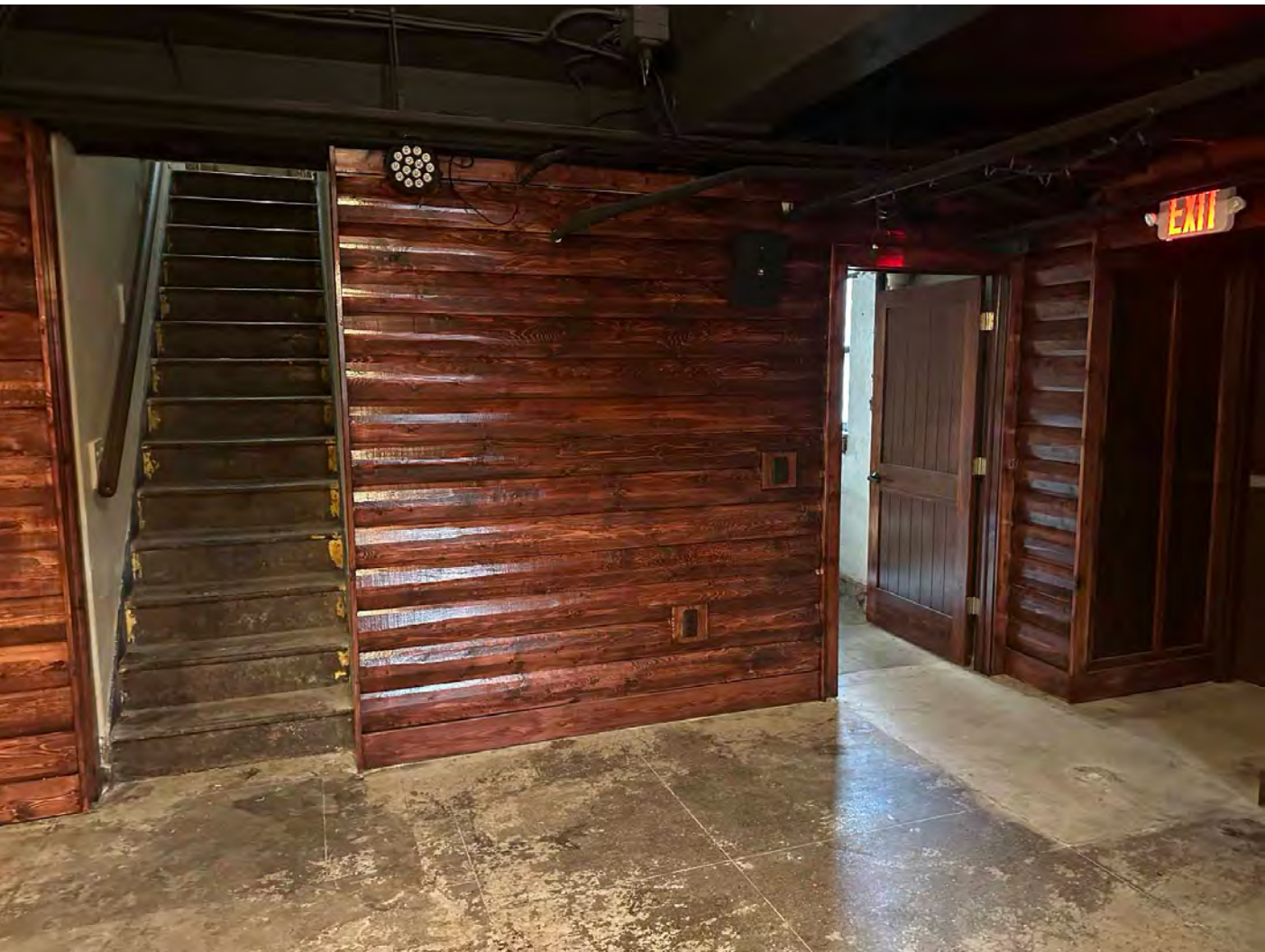
4 VIEW 4 A5.1 View up existing stairs towards proposed new stair location from basement
