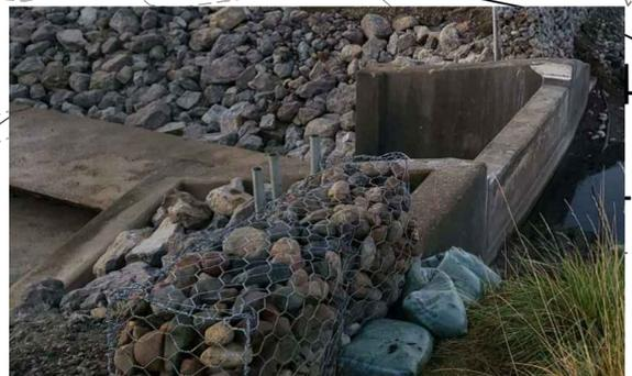
GABION BASKET: 5-FEET LONG, 15" WIDE X 36" TALL (0.70 CYD) 4 GA WIRE, FILLED WITH 3" TO 8" STONE. STRIP TOPSOIL, INSTALL ON GEOTEXTILE FABRIC AND COMPACTED CLAY USING POSTS SPACED AT 1-FOOT MAX.
