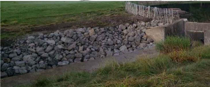
MDOT RIP RAP 8" X16" (NATURAL FIELD STONE OR ROCK - NO BROKEN CONCRETE) ON TOP OF GEOTEXTILE FABRIC, SLOPE SHALL NOT EXCEED 1:2 SLOPE; FILL ALONG BANK BETWEEN THE WEIR AND BRIDGE (10 CYD)
