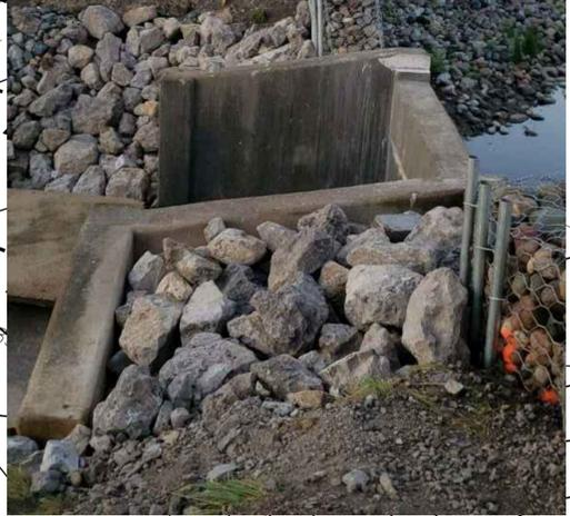
MDOT RIP RAP 8" X16" (NATURAL FIELD STONE OR ROCK - NO BROKEN CONCRETE) ON TOP OF GEOTEXTILE FABRIC, SLOPE SHALL NOT EXCEED 1:2 SLOPE; FILL ALONG BANK BETWEEN THE WEIR AND BRIDGE (1 CYD)
