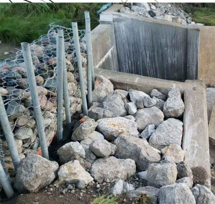
MDOT RIP RAP 8" X16" (NATURAL FIELD STONE OR ROCK - NO BROKEN CONCRETE) ON TOP OF GEOTEXTILE FABRIC, SLOPE SHALL NOT EXCEED 1:2 SLOPE; FILL ALONG BANK BETWEEN THE WEIR AND BRIDGE (1 CYD)
