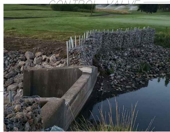
GABION BASKET: 25-FEET LONG, 15" WIDE X 36" TALL (3.5 CYD) 4 GA WIRE, FILLED WITH 3" TO 8" STONE. STRIP TOPSOIL, INSTALL ON GEOTEXTILE FABRIC AND COMPACTED CLAY USING POSTS SPACED AT 1-FOOT MAX.
