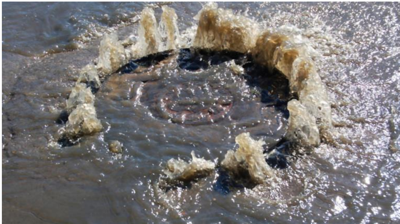
Sanitary Sewer Overflows
