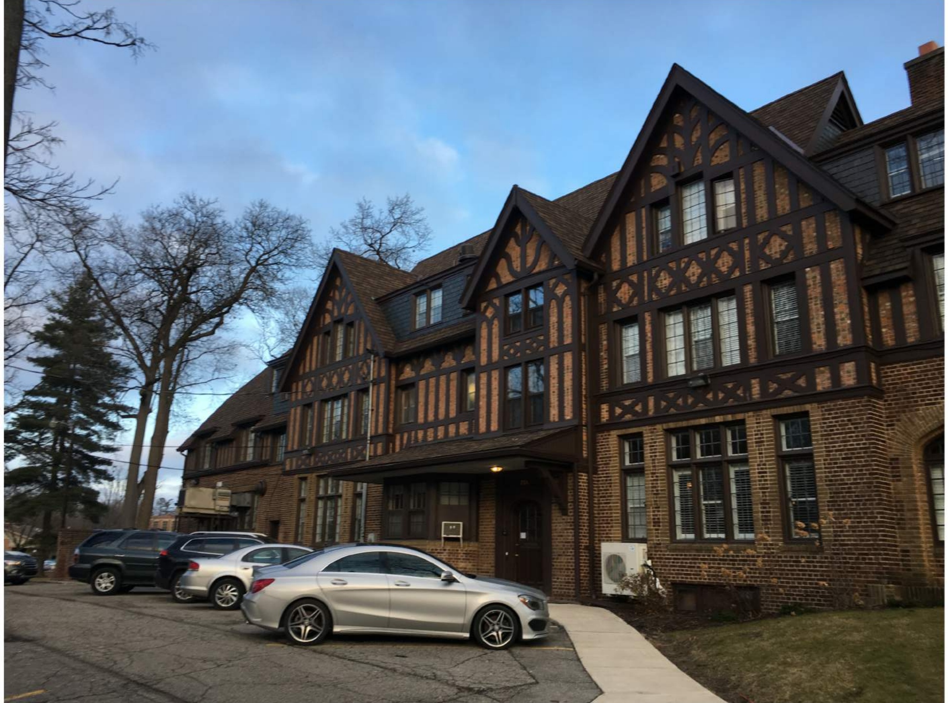
EXISTING SOUTHWEST CORNER OF BUILDING
