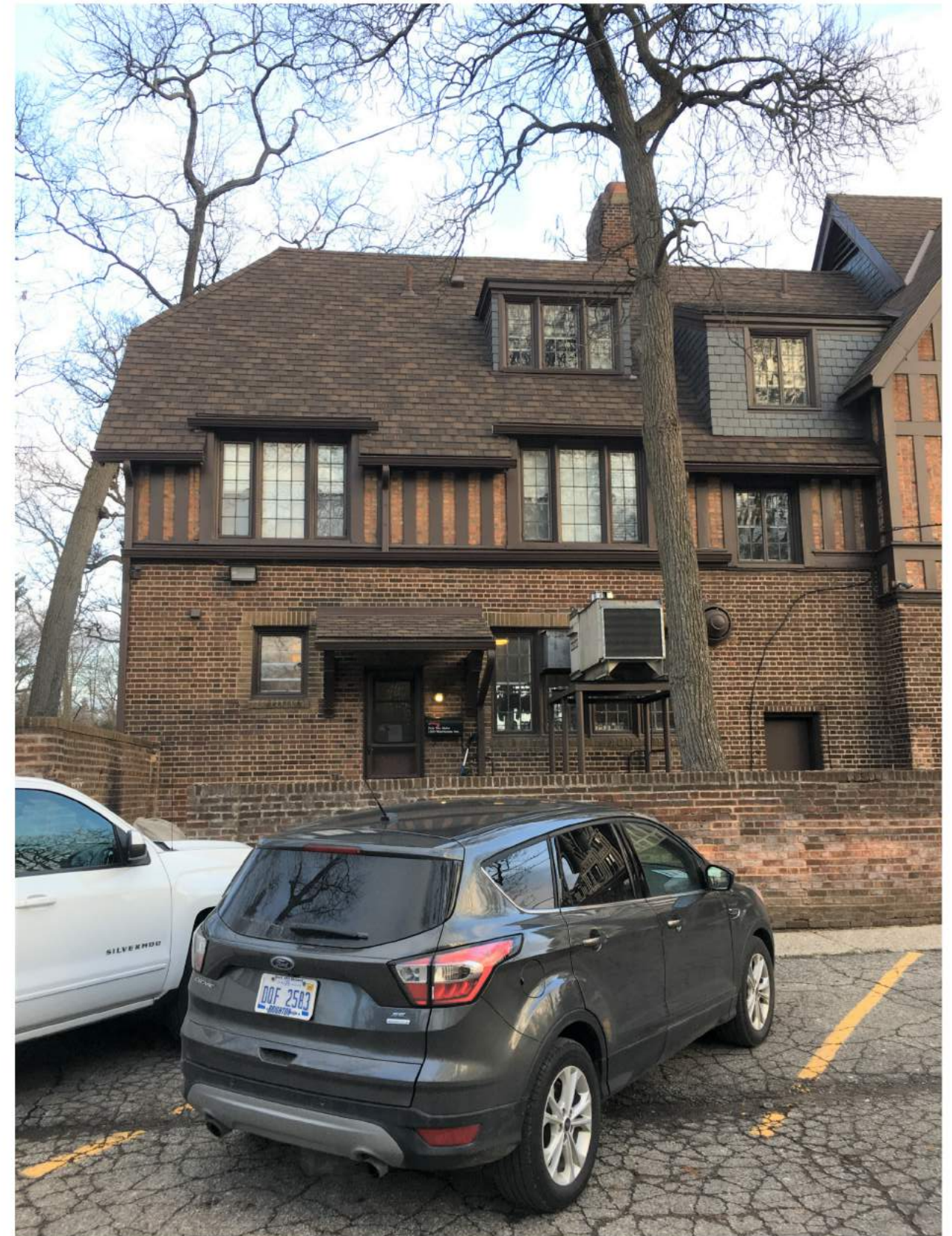
EXISTING NORTHWEST CORNER OF BUILDING
