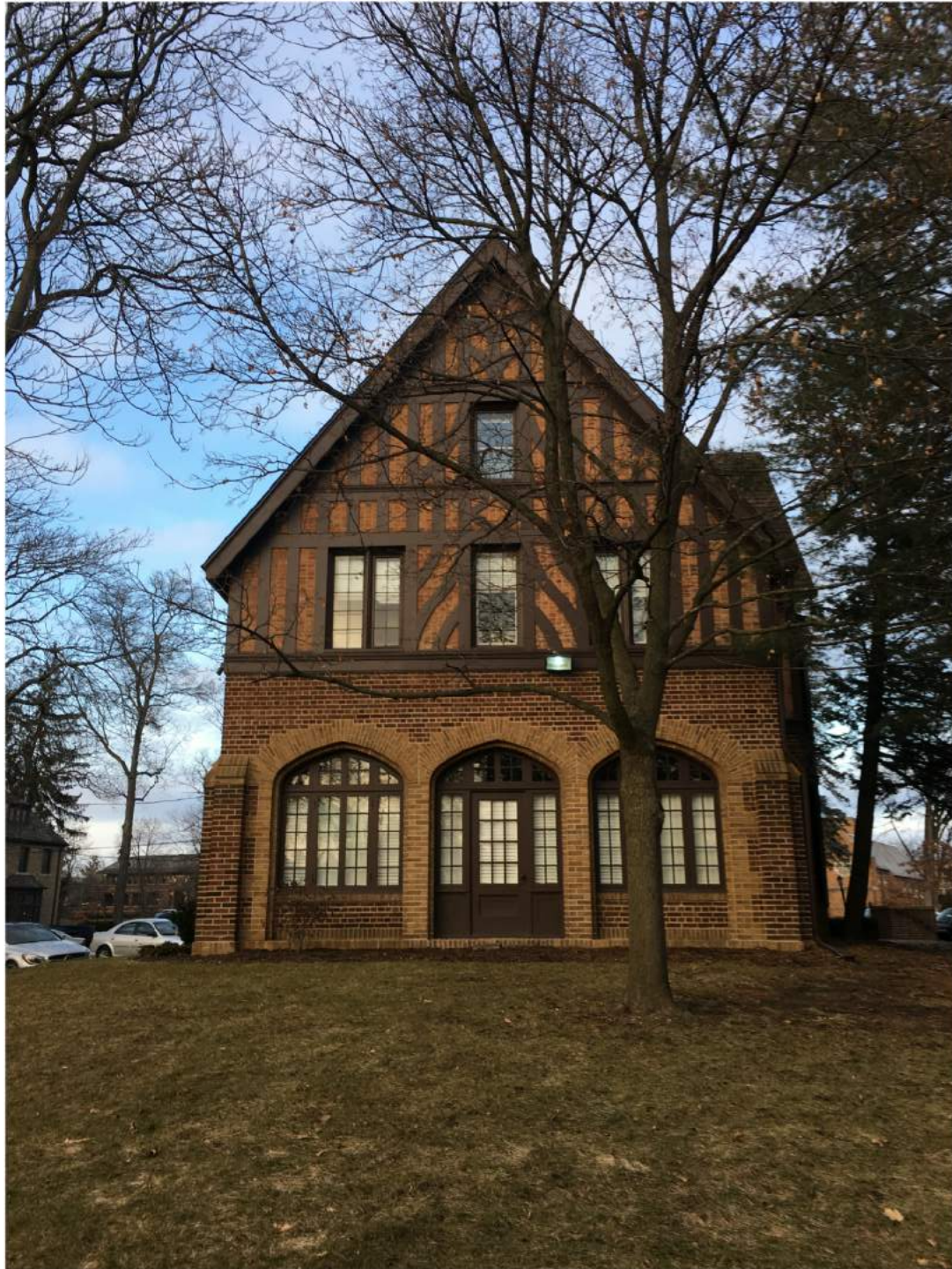
EXISTING SOUTH SIDE OF BUILDING
