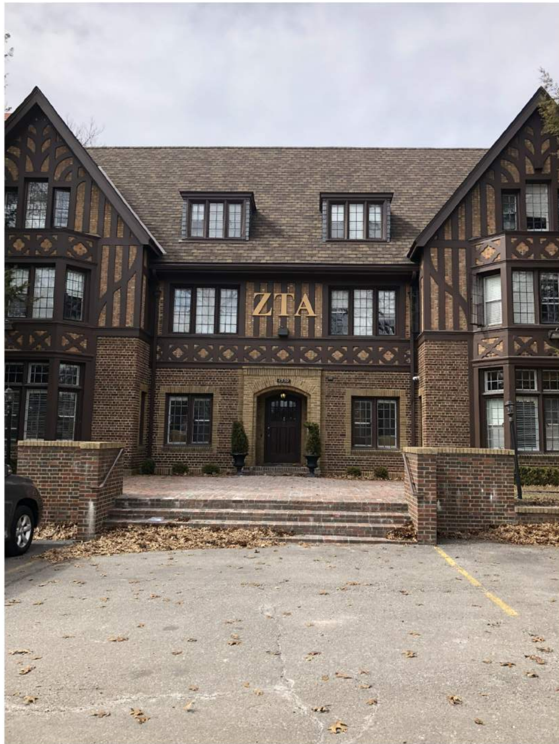
VIEW OF FRONT ENTRANCE
