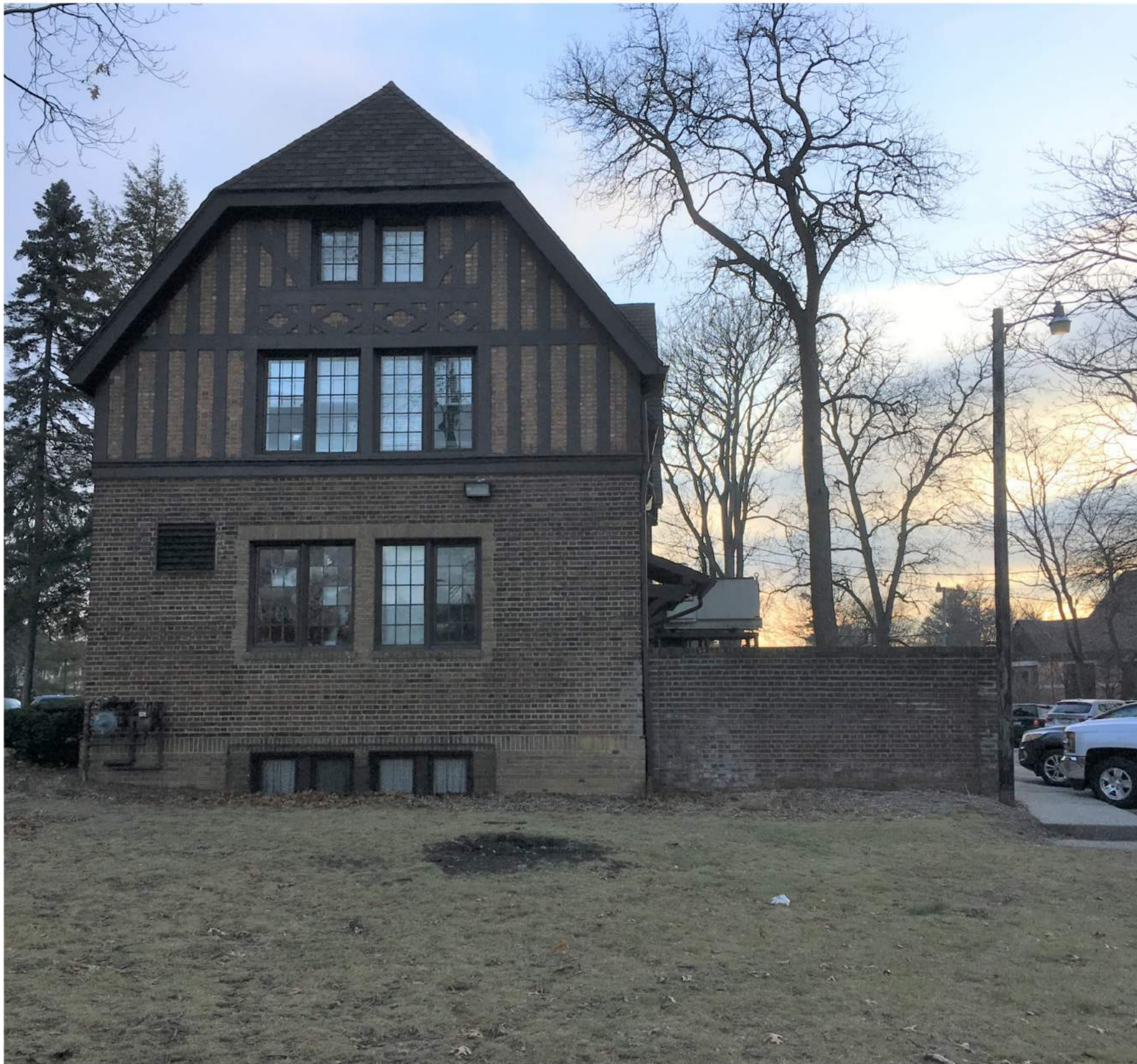
EXISTING NORTHWEST CORNER OF BUILDING
