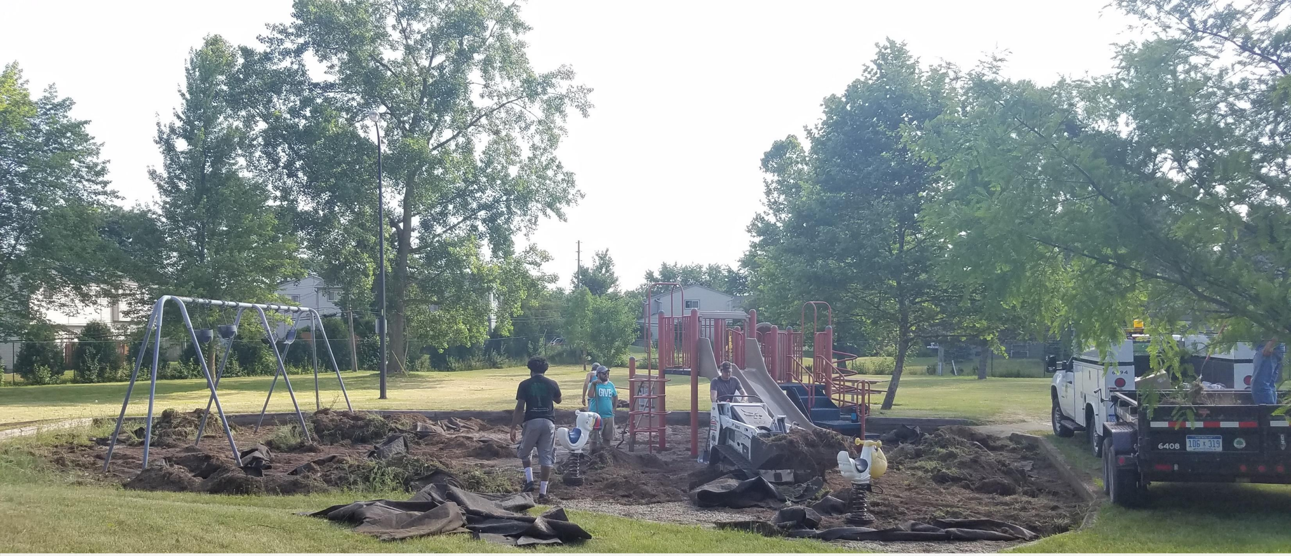
Digging out and removing top layer
