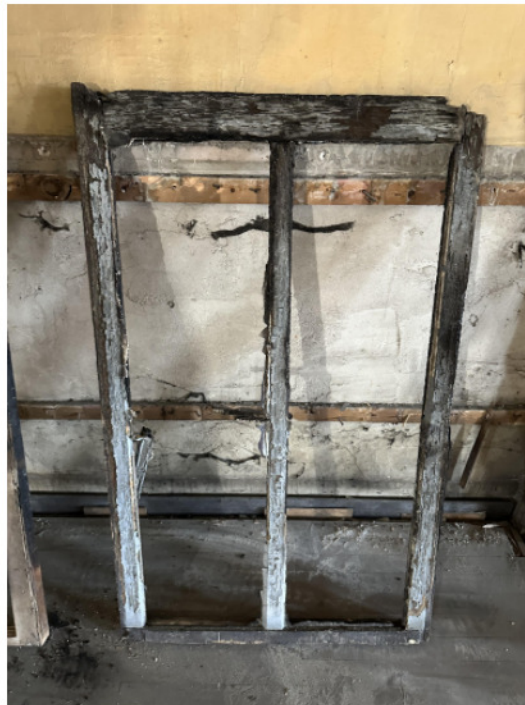
1 (E) WINDOW MULLIONS FIRE DAMAGE N.T.S.
