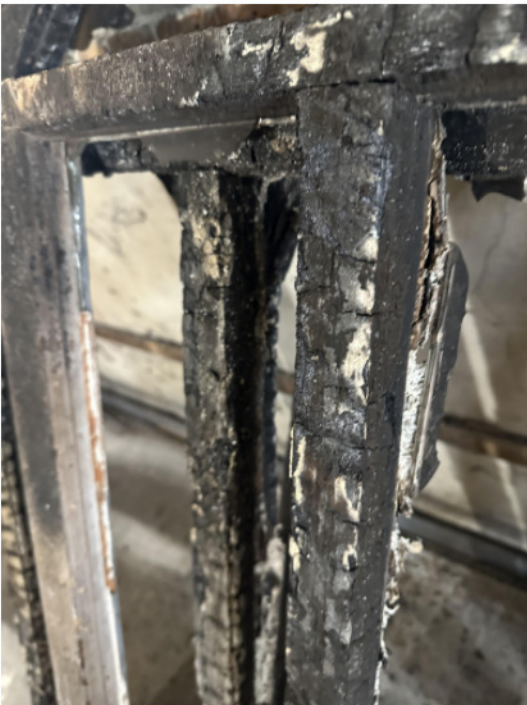
1 (E) WINDOW MULLIONS FIRE DAMAGE N.T.S.
