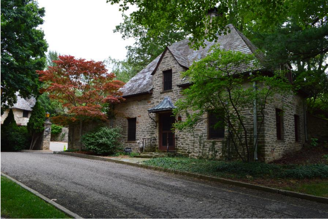
5 - Looking northeast at gardener's cottage with house to left, July 2017
