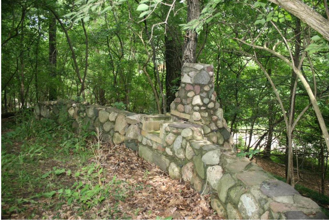
15 - Fireplace built into east wall of wild garden, July 2017
