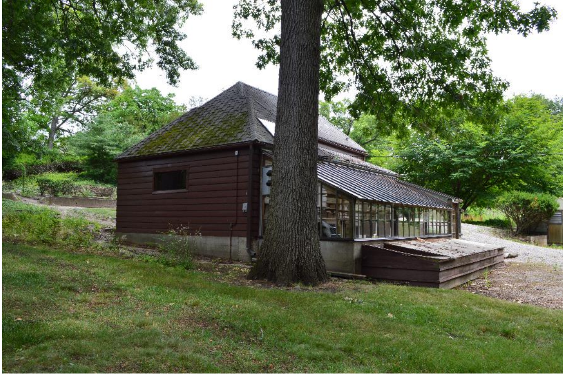
7 - Looking northeast at shop and greenhouse, July 2017
