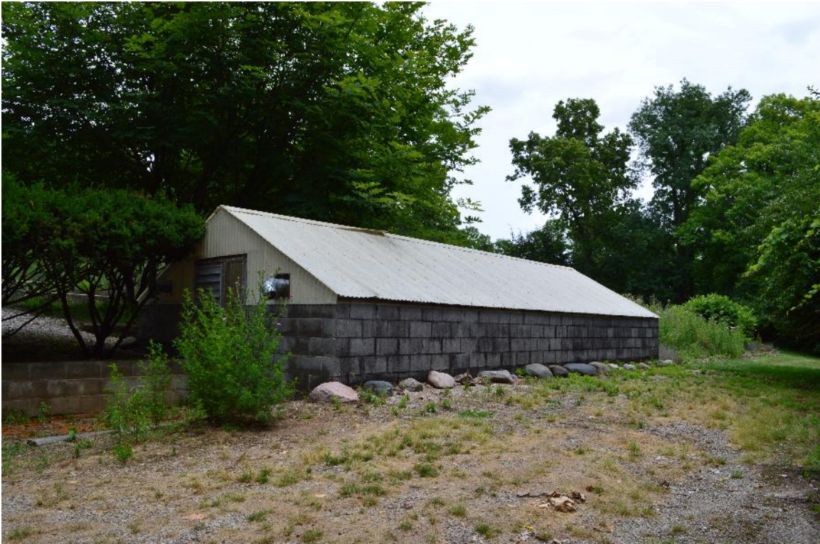
10 - Looking northeast at coldhouse, July 2017
