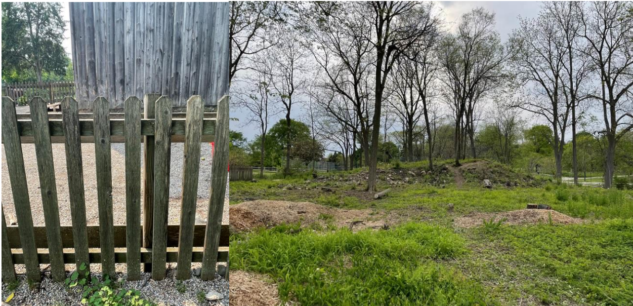
Existing picket fence around animal barn. Dimensions and design of new fencing will match this existing design on the property.
