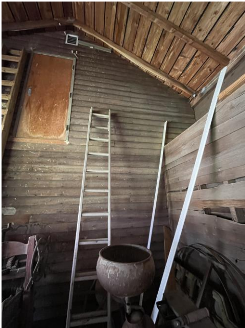
Interior south wall of woodshed. The ladder egress will be replaced with a stairwell. The existing loft (above the hallway bump-out in photo) will be extended.
