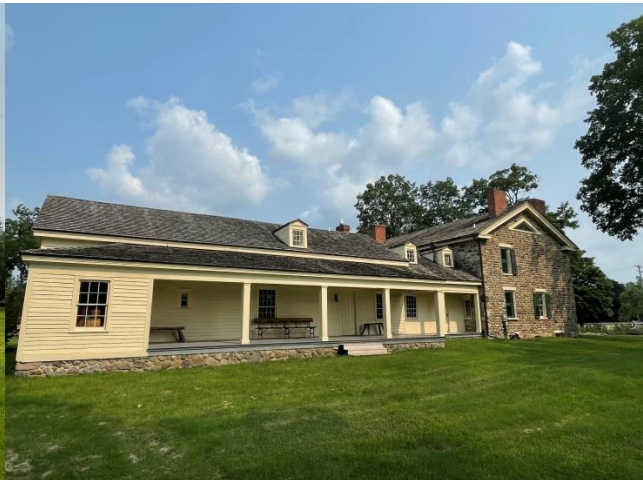
West porch of farmhouse.
