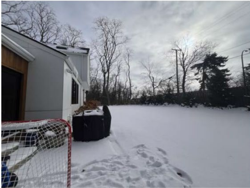
View of Fence from Rear Yard
