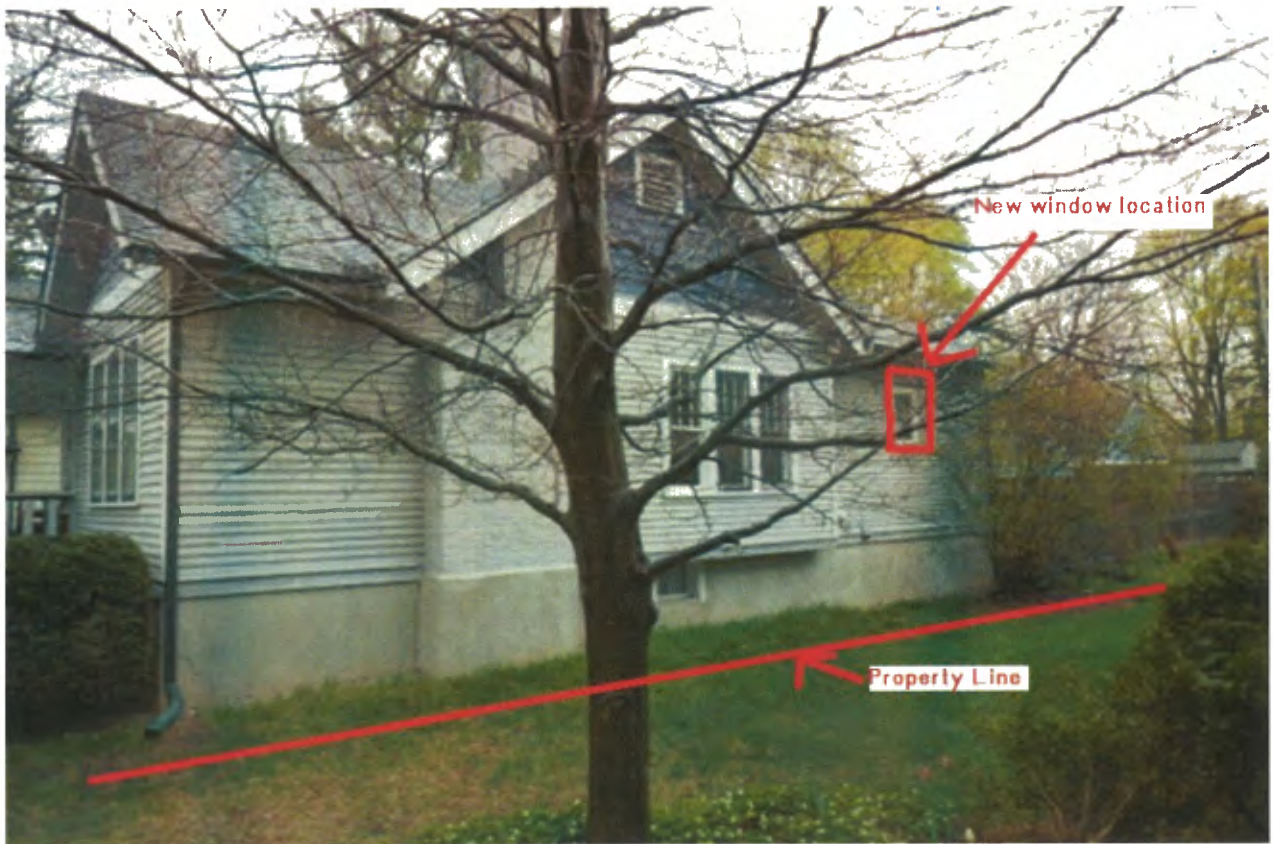
View of west side of house showing proposed location of new 1 hour window.
