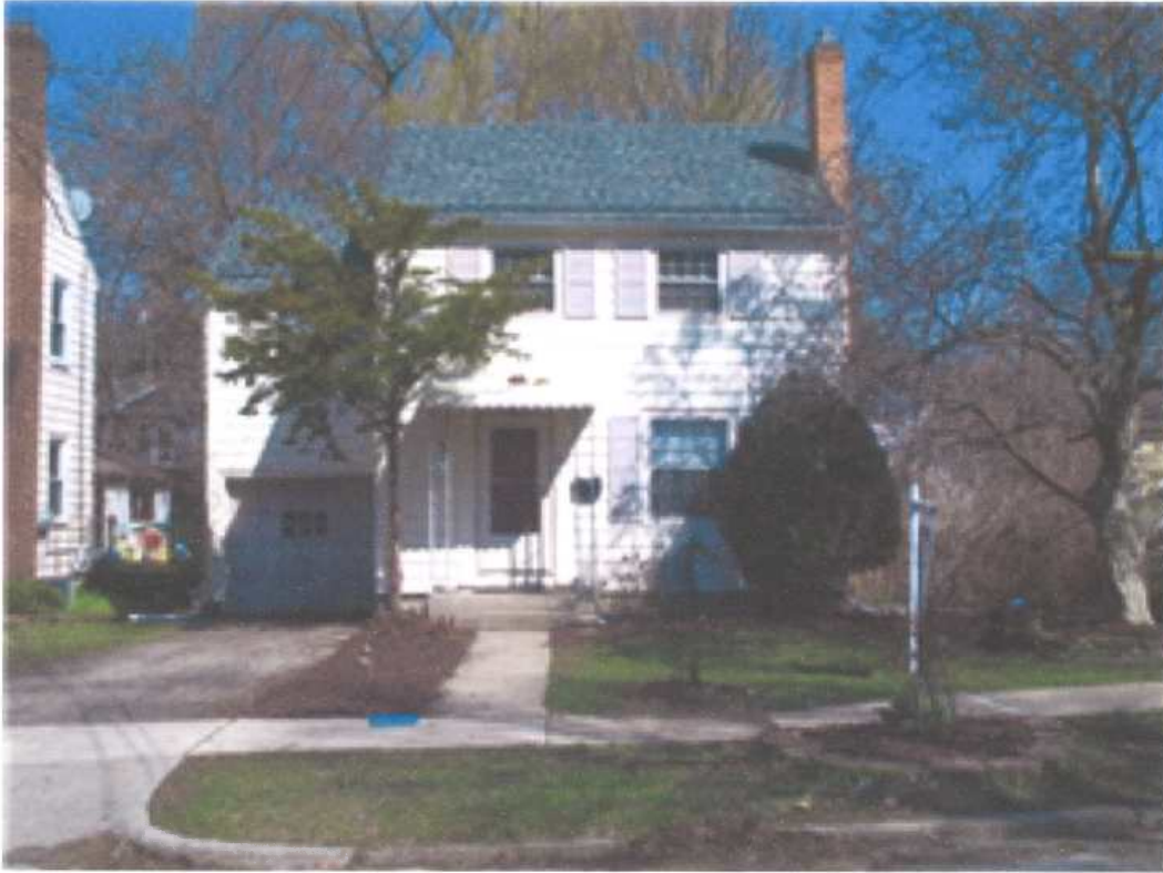
500 Maple Ridge, West Elevation
