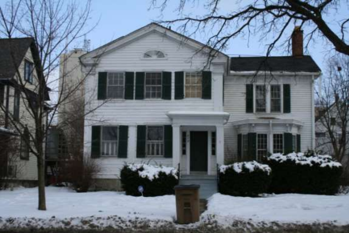
Photograph 6 – 415 South Fifth Avenue, Gaskell/Beakes House, February 2010
