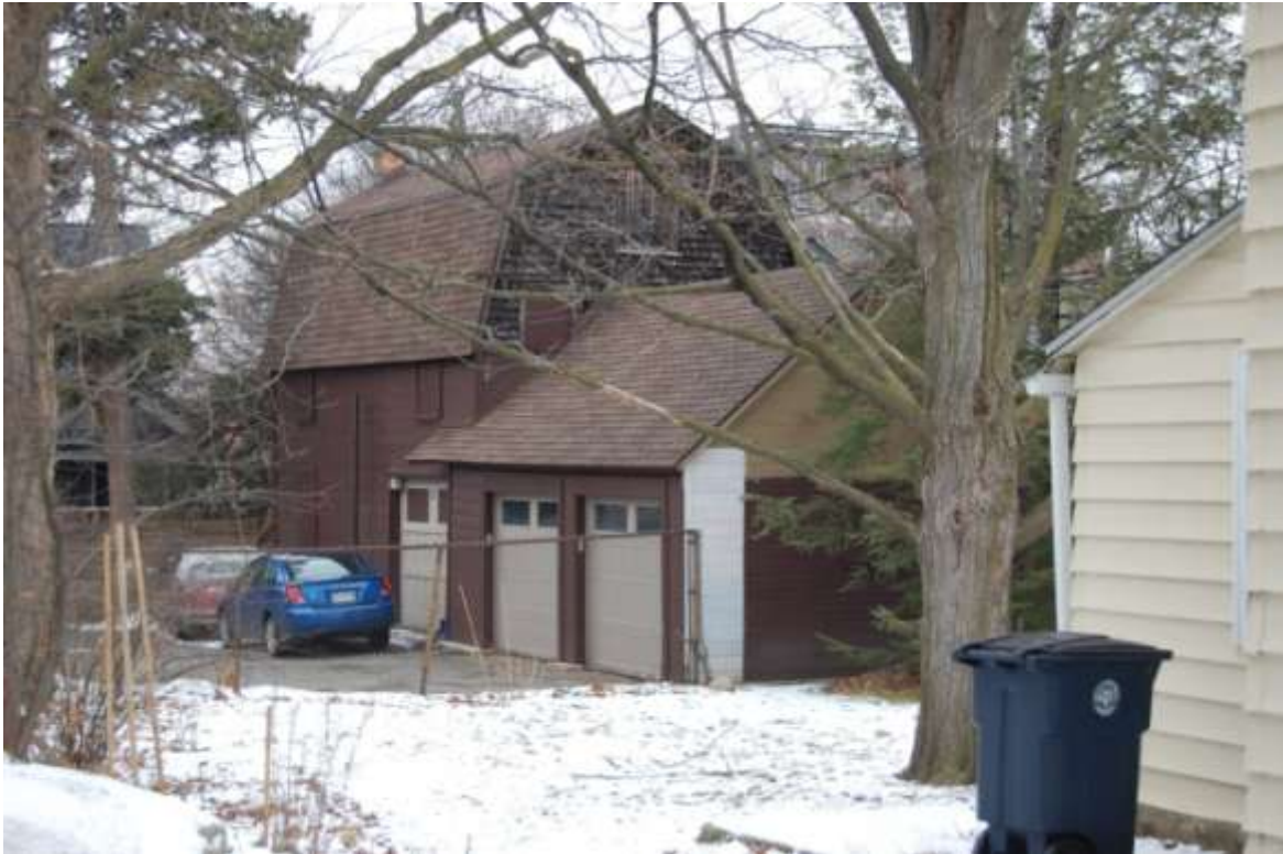
Photograph 14 – Barn at 215 Packard Street, February 2010
