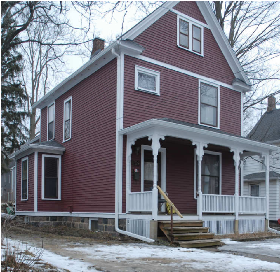
808 West Washington Street - Side elevation (west)
