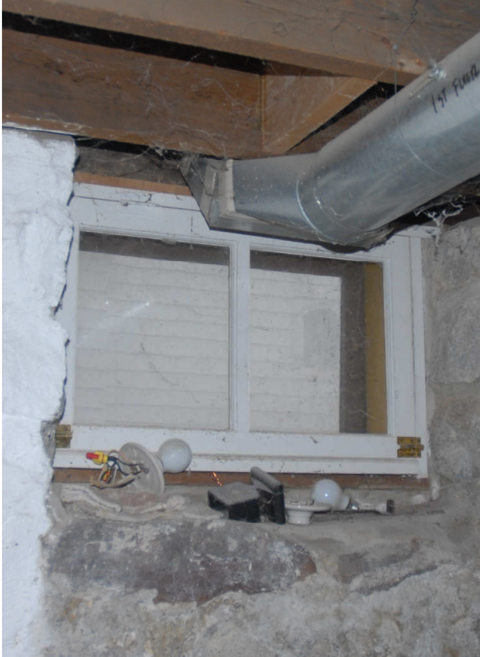
basement window # B2
