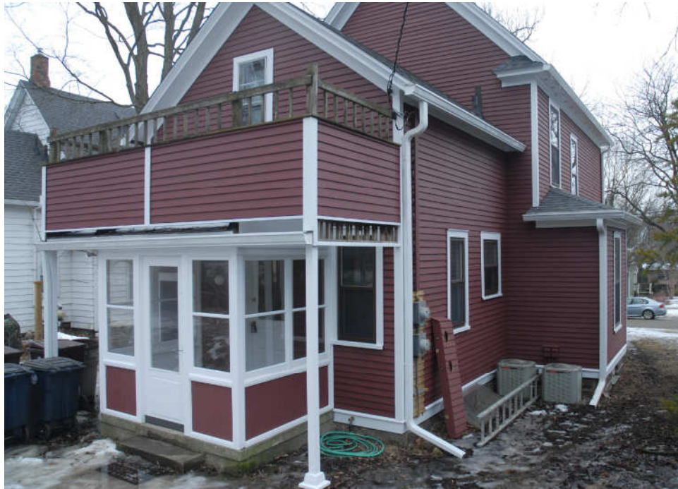
808 West Washington Street - Side elevation (west)
