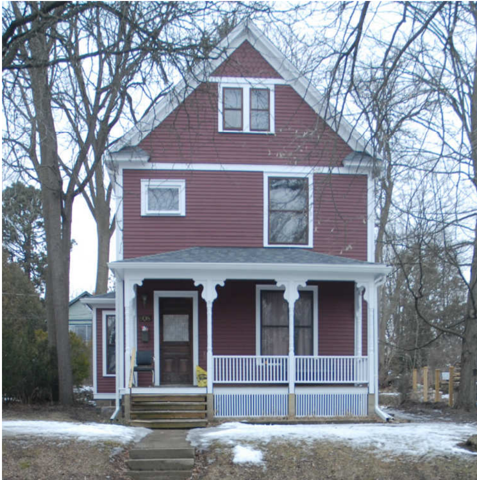
808 West Washington Street - Front elevation (south)
