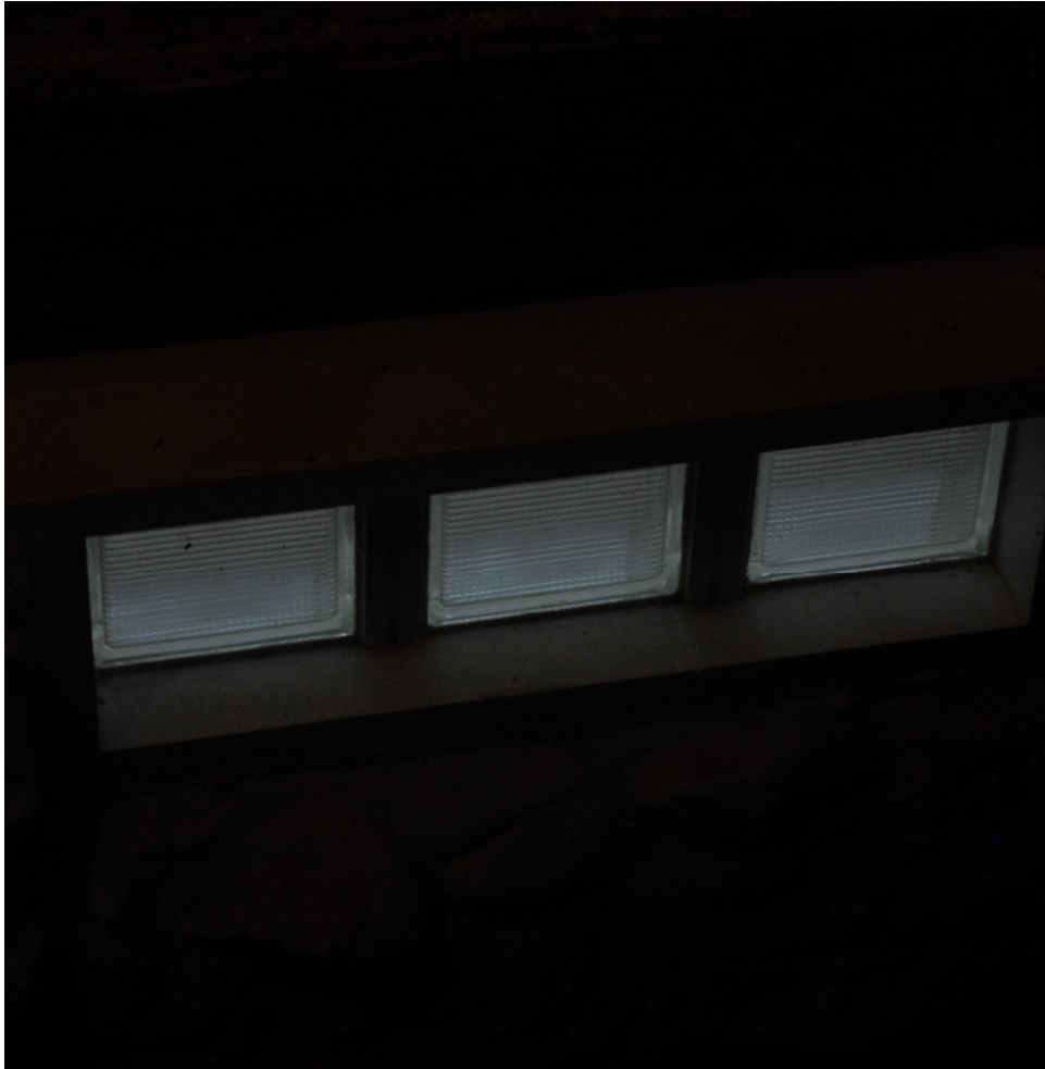
basement window # B1
