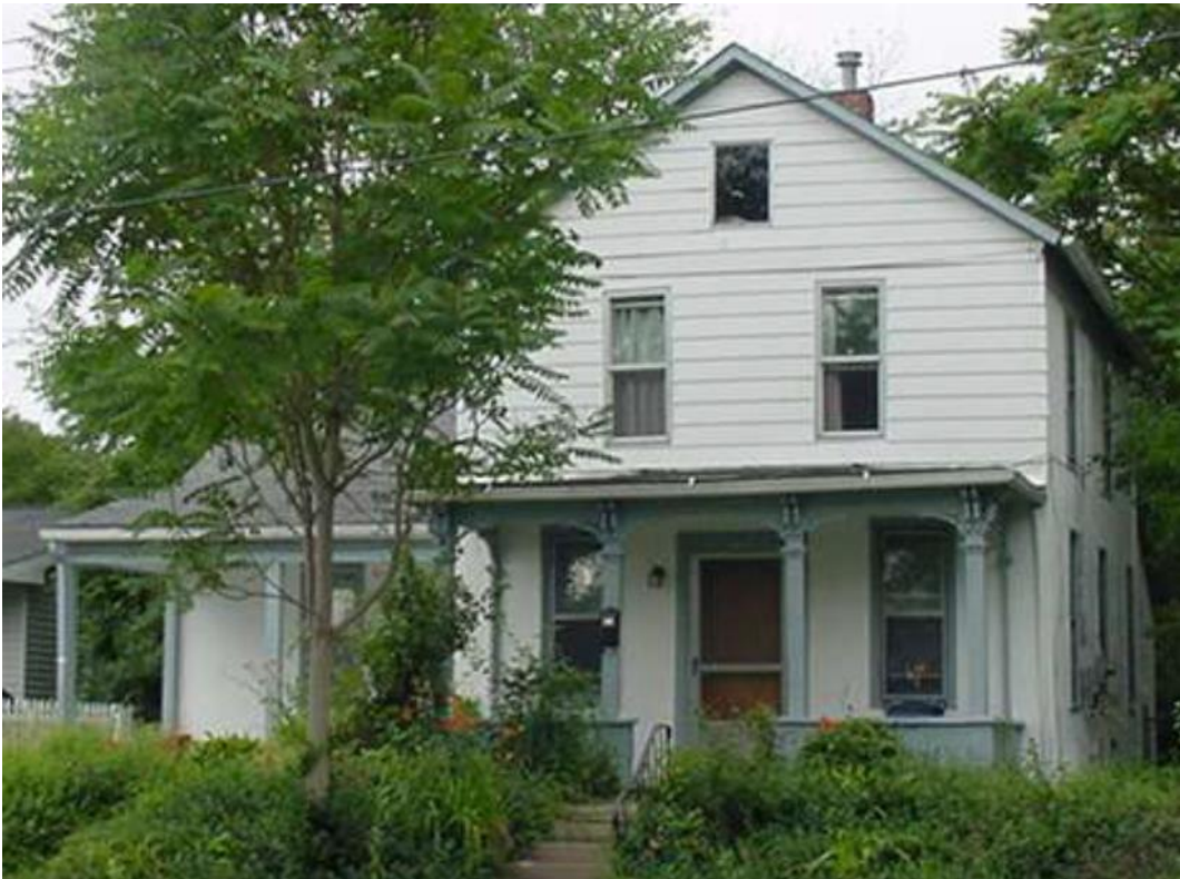
1137 Traver Road (2007 survey photo)
