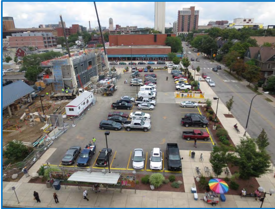
View from Fourth & William Parking Structure
