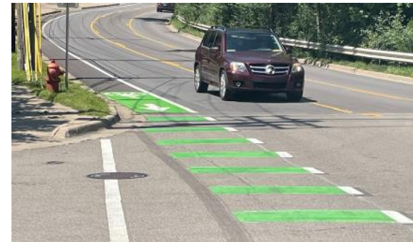
Intersection Conflict Markings
