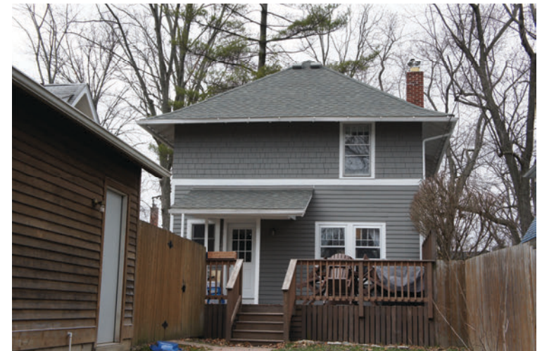
photo right: Rear (east elevation). the non historic porch will be removed to accommodate the new rear addition. One original window on the second floor will be removed. Two original windows on the first floor will be reused in the new second floor addition.
