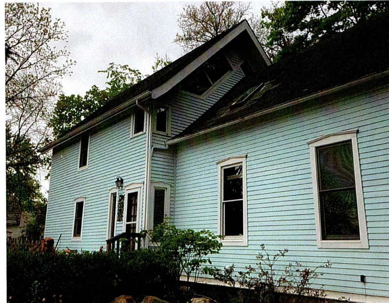
NORTH ELEVATION: NEW KITCHEN WINDOW AT THE REAR OF THE HOUSE, NEW WINDOW IN BEDROOM (MATCH EXISTING SIZE AND STYLE OF EXISTING)
