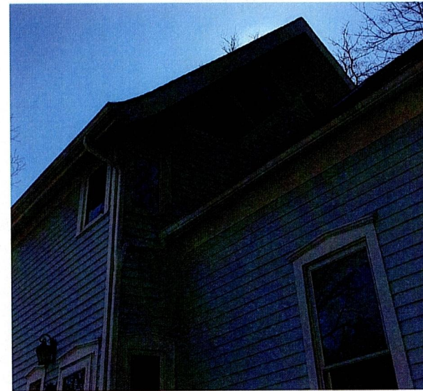
WEST ELEVATION (STREET FACING): NEW FIXED, DOUBLE-PANE WINDOWS IN LOCATION OF EXISTING 2ND FLOOR ANGLED AWNING WINDOWS
