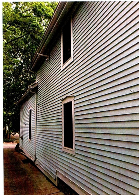
SOUTH ELEVATION (LOOKING WEST): NEW WINDOWS AT REAR OF HOUSE, NEW TEMPERED WINDOW IN ENTRY TO MATCH EXISTING KITCHEN WINDOW
