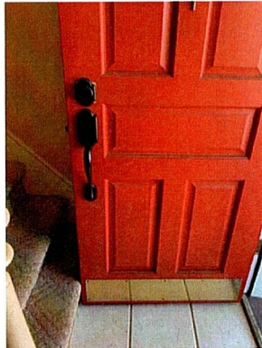
36" ENTRY DOOR CANNOT FULLY OPEN
