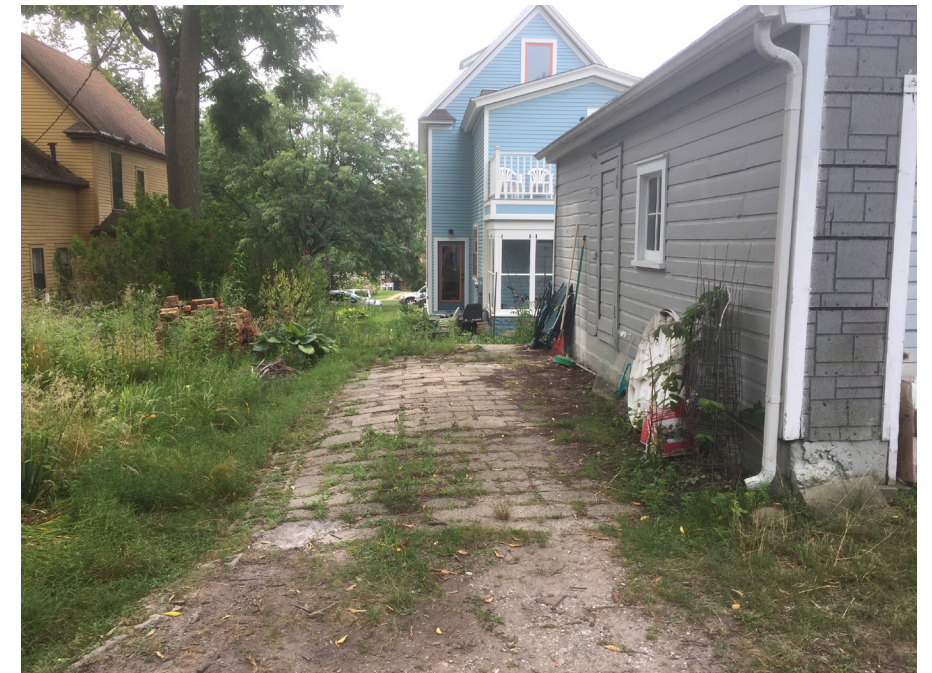
Existing cinder block parking spur, proposed removal and 4' wide pathway along garage with increased planting area.
