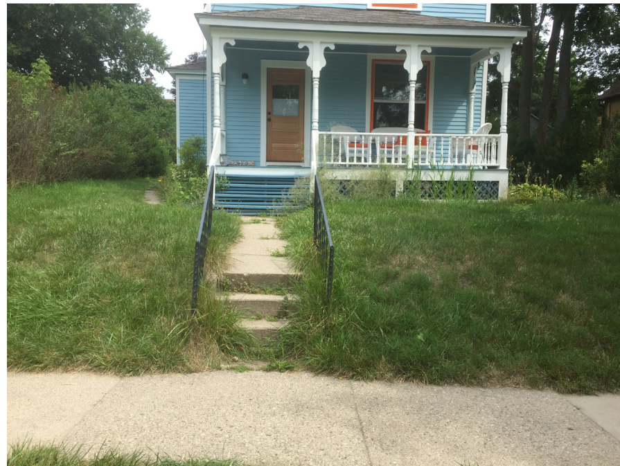
Existing steps from sidewalk to front door, proposed widening to 6' width of porch steps.
