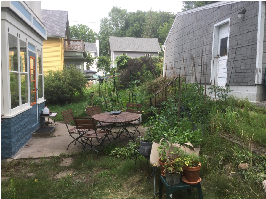
Existing steps from back of house to upper level garage, cinder block retaining walls buried behind vegetation.
