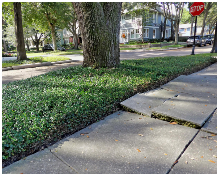
Figure 2. Sidewalk damage caused by a large southern live oak ( Quercus virginiana ). Credits: Deborah R. Hilbert, UF/IFAS
