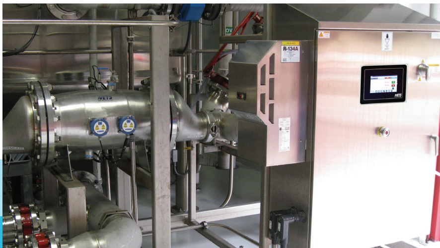
ETS-UV generator - ECF model with Spectra Touch Controller inside a NEMA 4X panel
