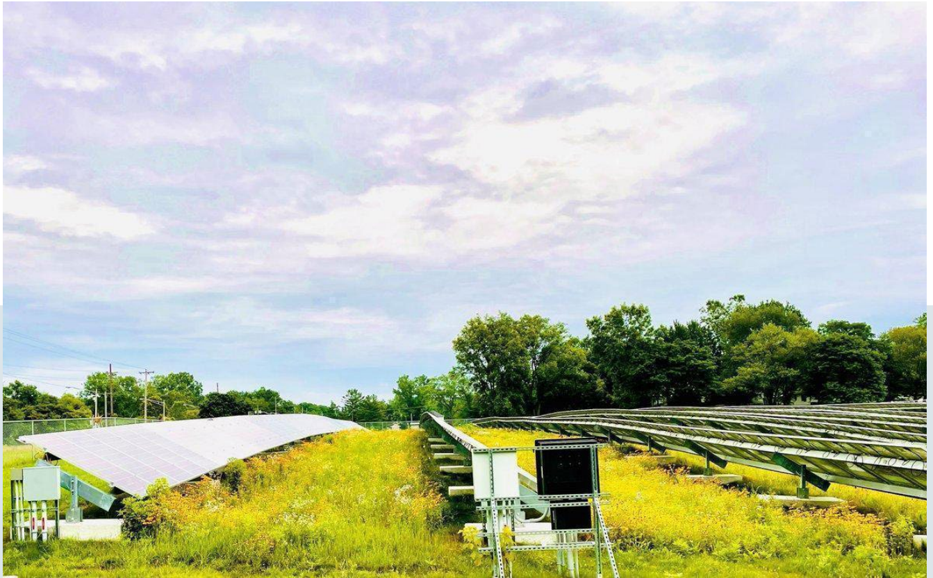
The East Lansing Community Solar Park.
